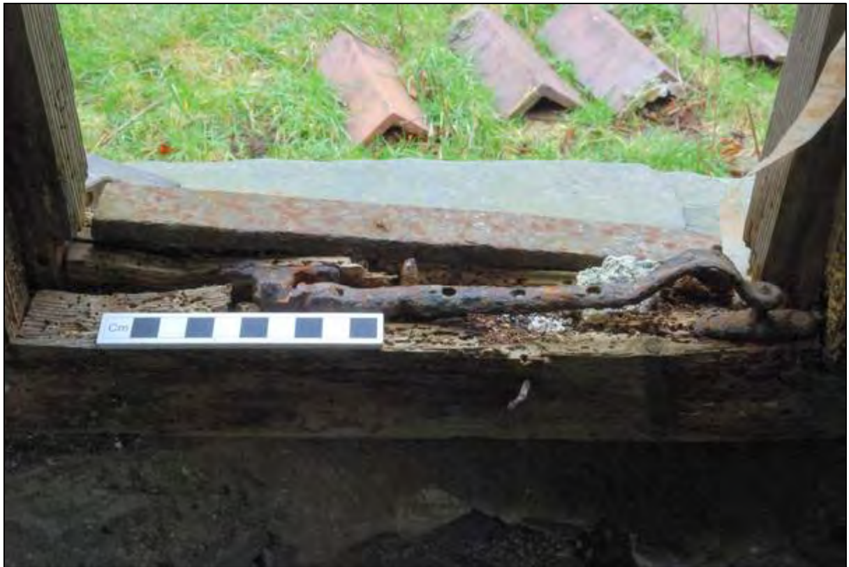
Plate 21: The latch lifter for the front window in the main room
