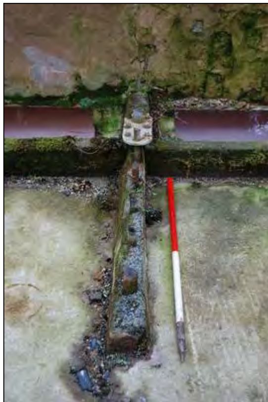
Plate 12: The divider between the bays in the cow house
