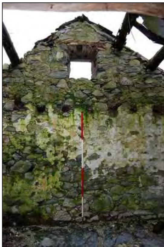
Plate 28: The supports for the croglofft and the upper window.
