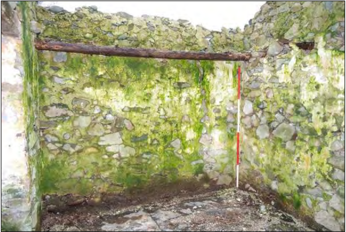
Plate 29: The surviving joist for the crogloff .
