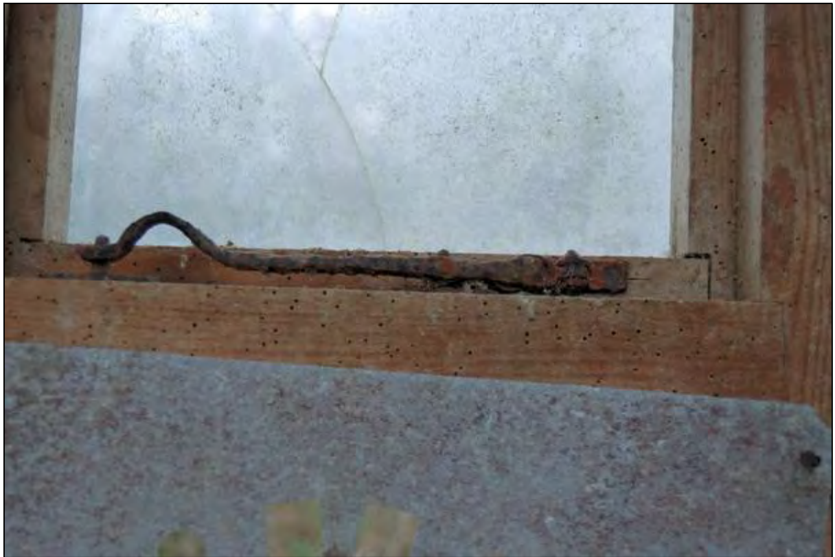
Plate 27: The latch lifter for the window in the bedroom
