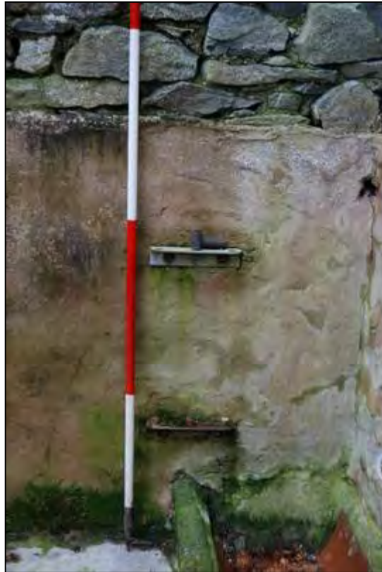
Plate 13: Fittings for the bars in front of the trough in the cow house
