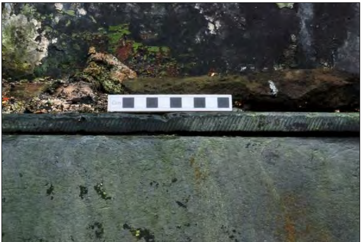
Plate 18: Detail of the slate surround showing the saw marks
