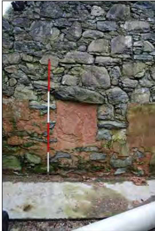
Plate 15: Blocked opening in the south eastern gable wall of the cottage
