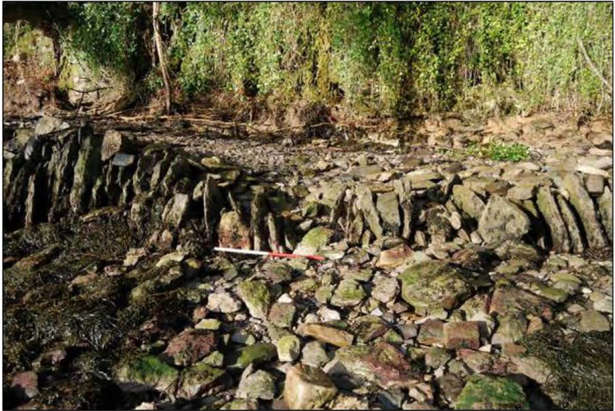
Plate 3: Possible slipway to the north of the pump house
