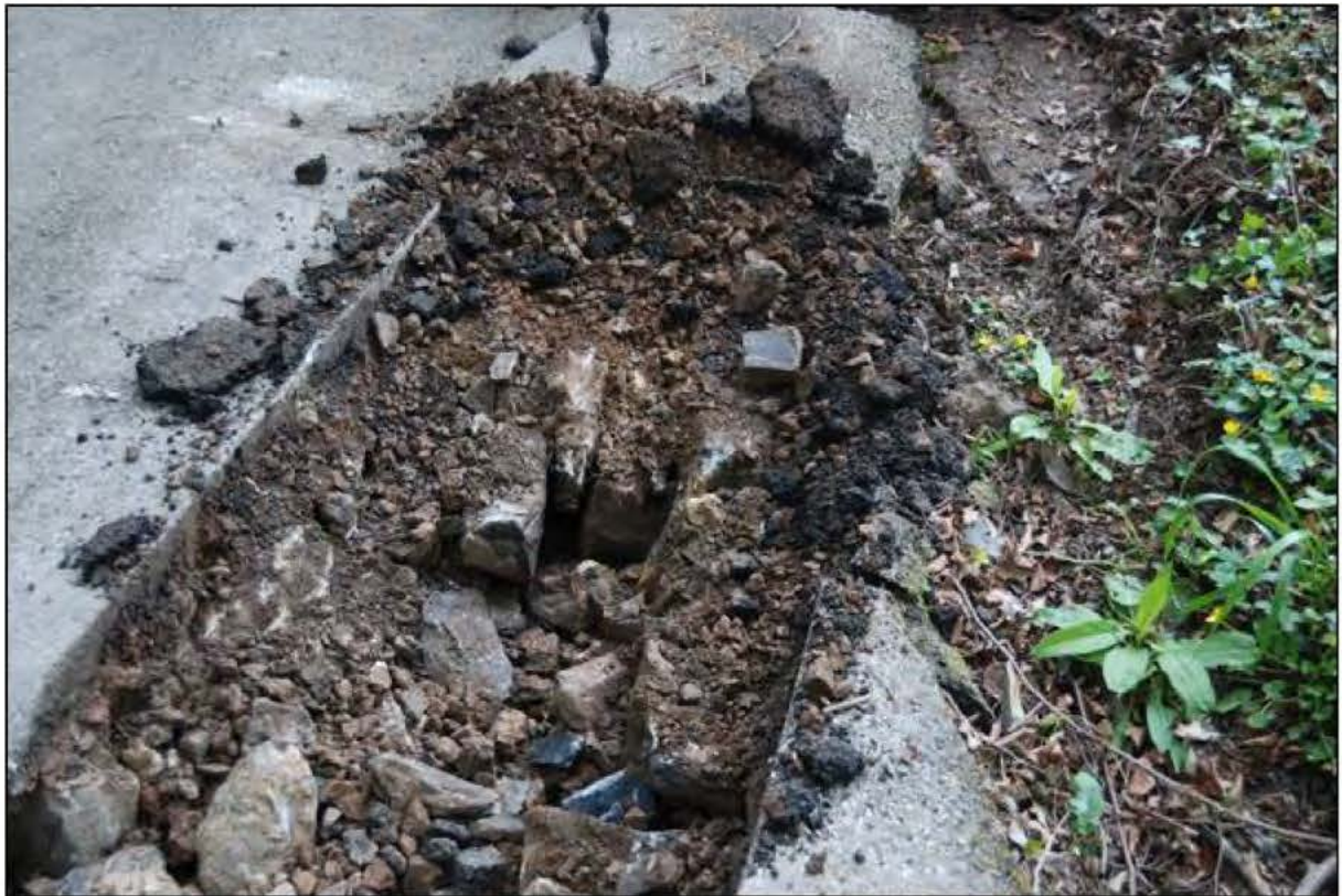
Plate 27: Pitched stones below the tarmac
