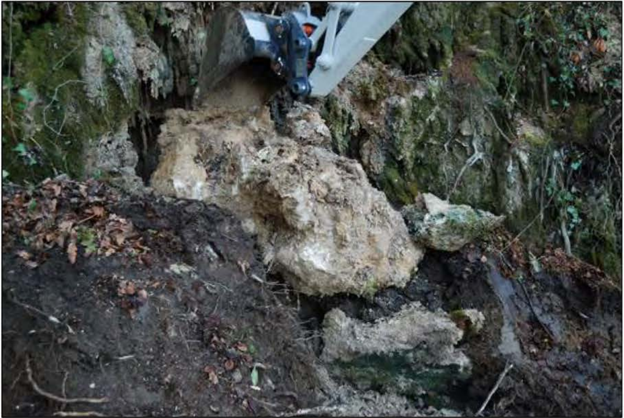
Plate 7: Removing the tufa from the cliff face
