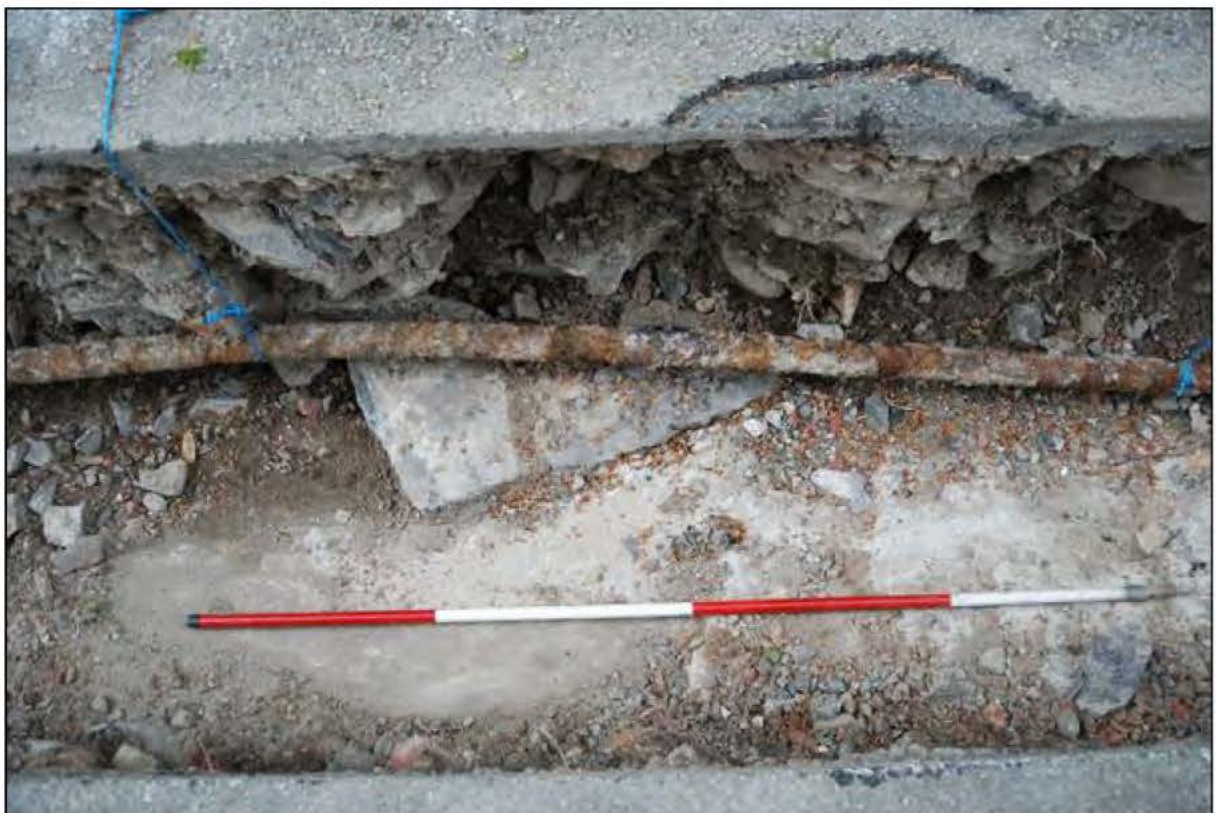
Plate 28: Concrete pad (Context 22)
