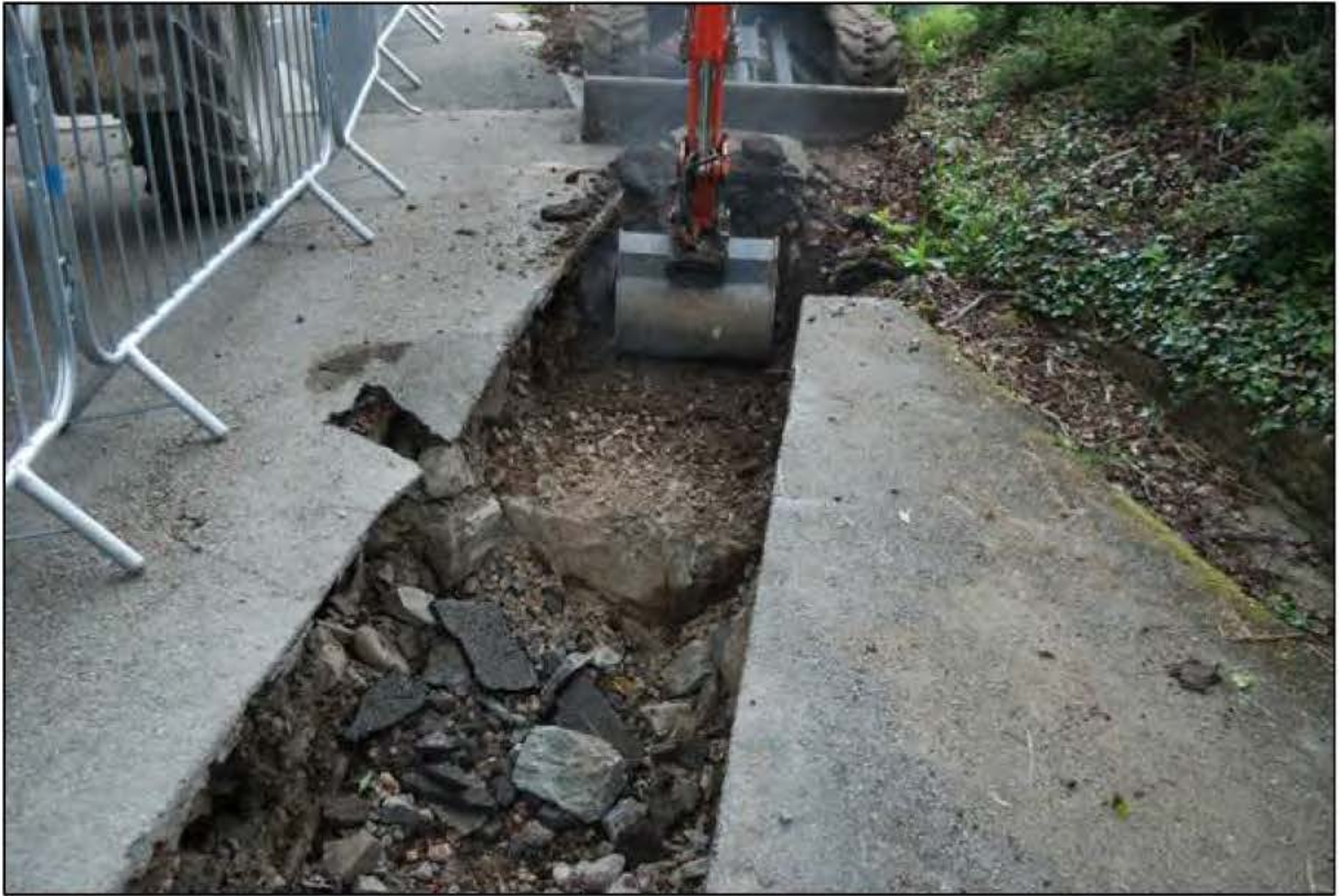
Plate 29: Step in the underlying limestone (Context 24)
