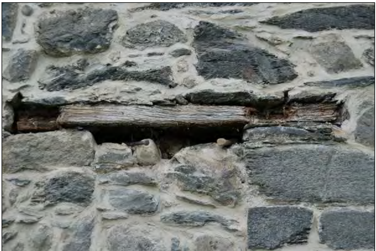
Plate 18: Lintel above the blocked doorway
