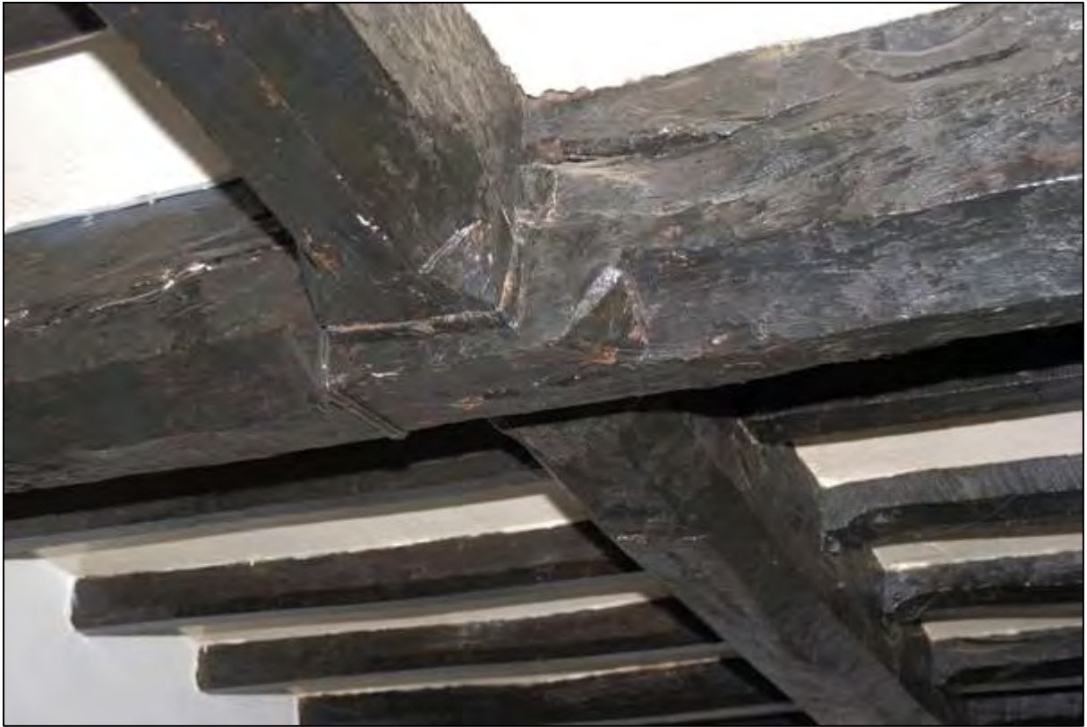
Plate 45: The boss between the transverse and one of the axial ceiling beams
