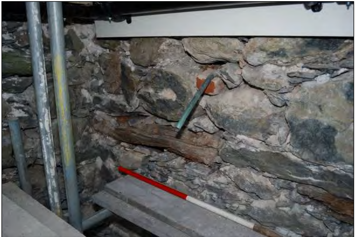
Plate 25: Detail of the lintel for the blocked window in the “Kitchen Range”
