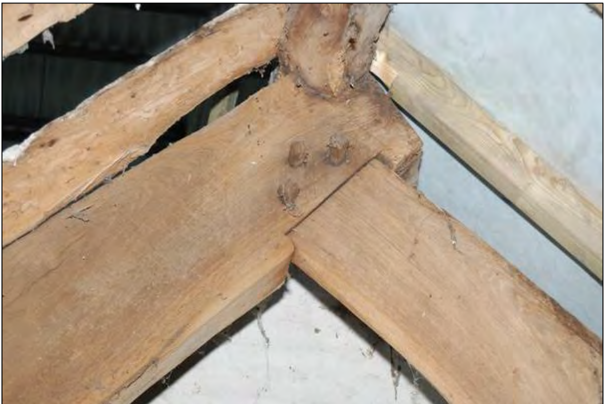
Plate 68: The peak of Truss 2 showing the notch for the ridge piece and the pegged joint between the principle rafters.
