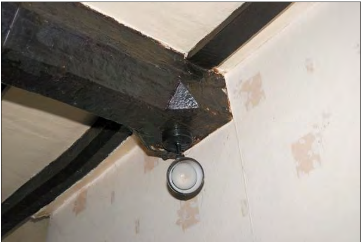
Plate 46: Straight cut stop on one of the axial beam in the hall
