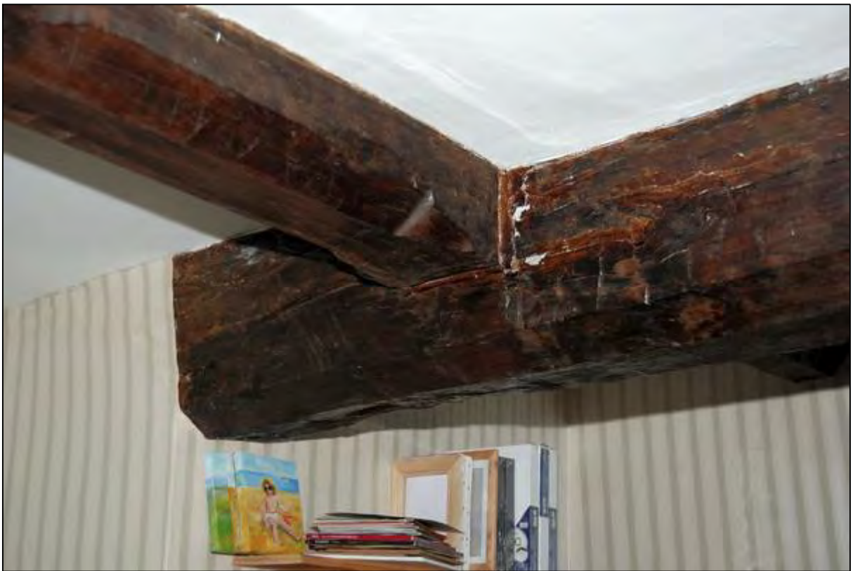
Plate 52: Rolled stops on one of the southern axial beams in the parlour
