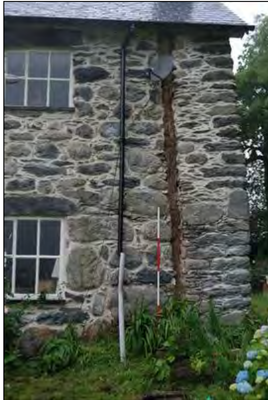
Plate 7: Wooden post exposed by the restoration works
