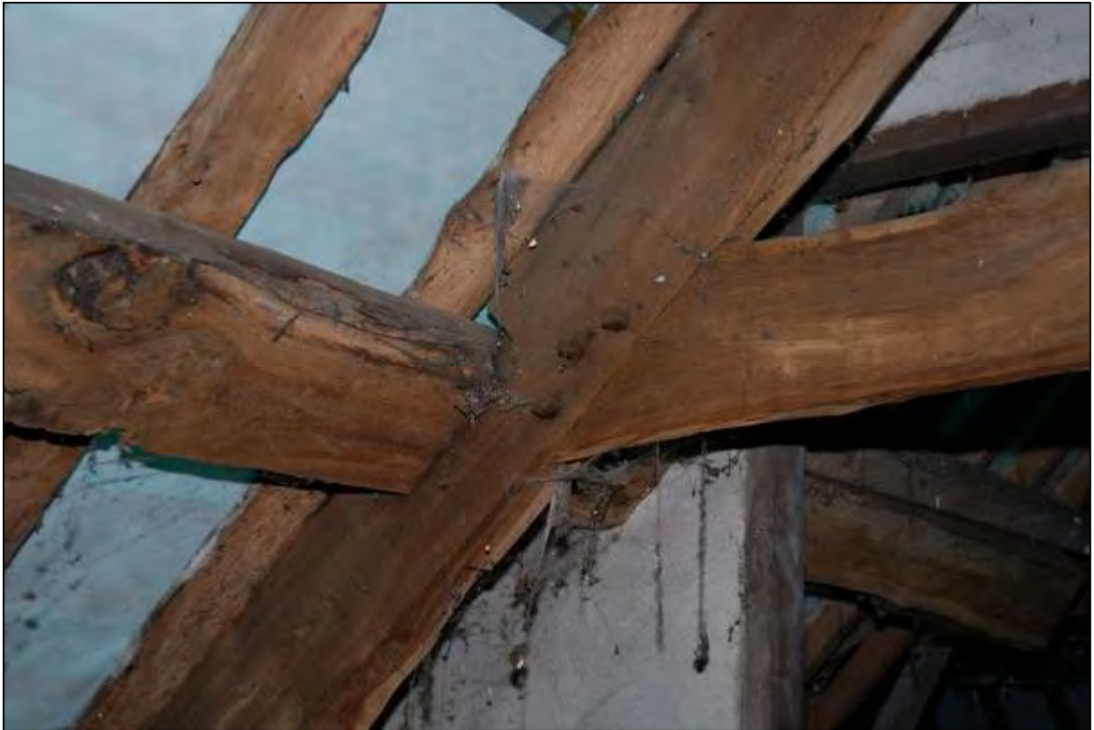
Plate 69: Trenching for the upper purlin
