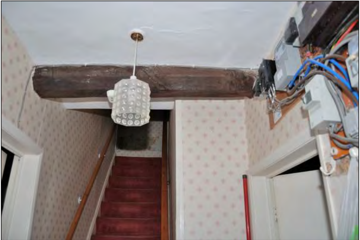
Plate 49: Axial Beal crossing the entrance hallway
