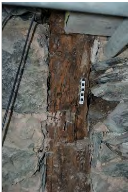
Plate 7: Wooden post exposed by the restoration works
