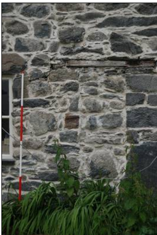
Plate 17: Blocked doorway in the front elevation
