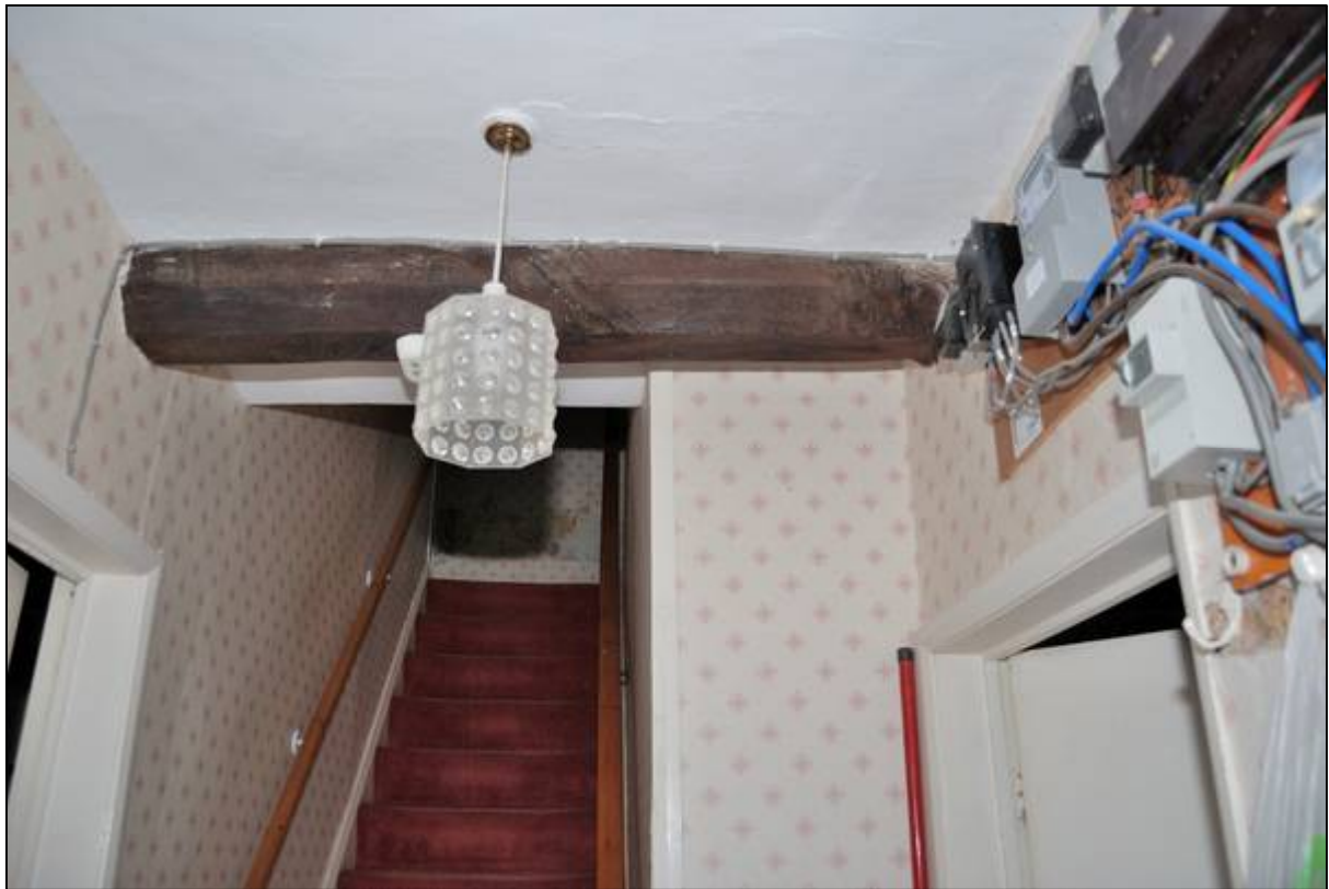
Plate 49: Axial Beal crossing the entrance hallway
