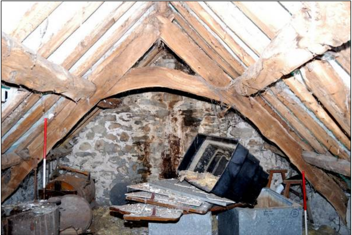
Plate 67: Truss 1, looking west
