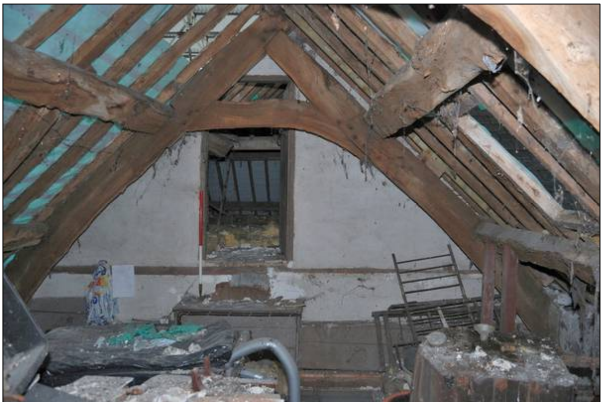
Plate 66: Truss 2 looking east
