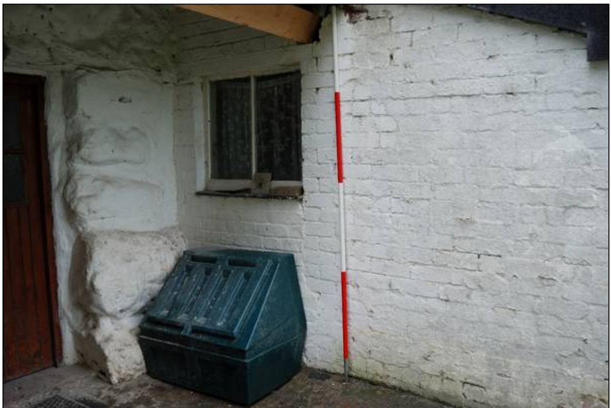
Plate 32: Blocked doorway in the scullery
