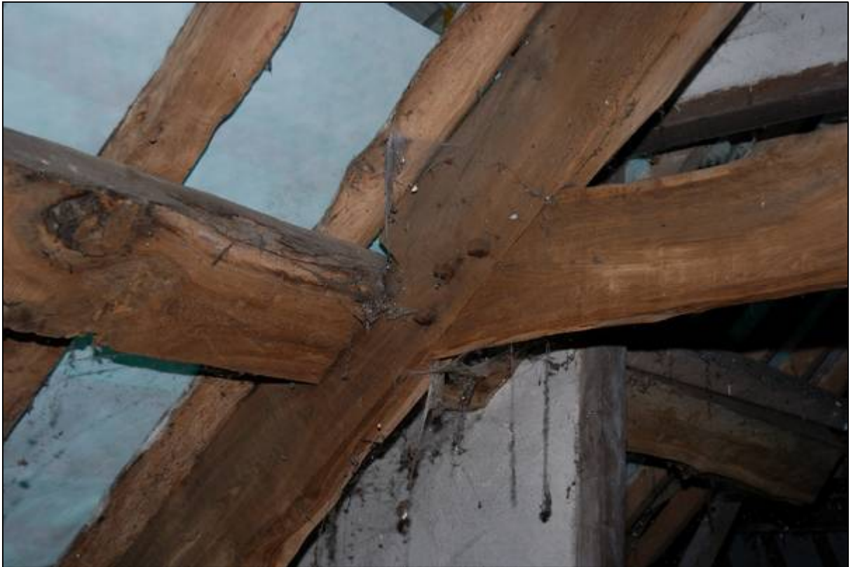
Plate 69: Trenching for the upper purlin
