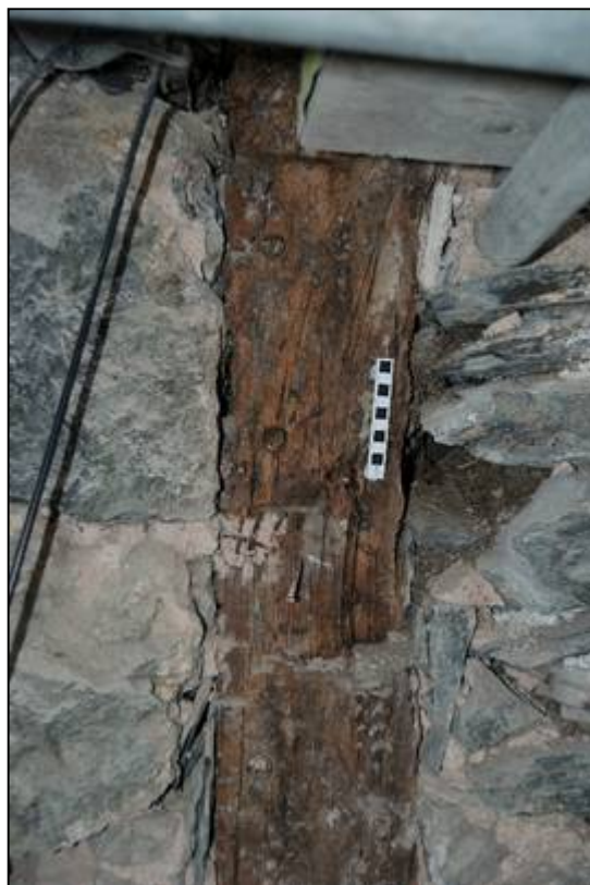
Plate 7: Wooden post exposed by the restoration works
