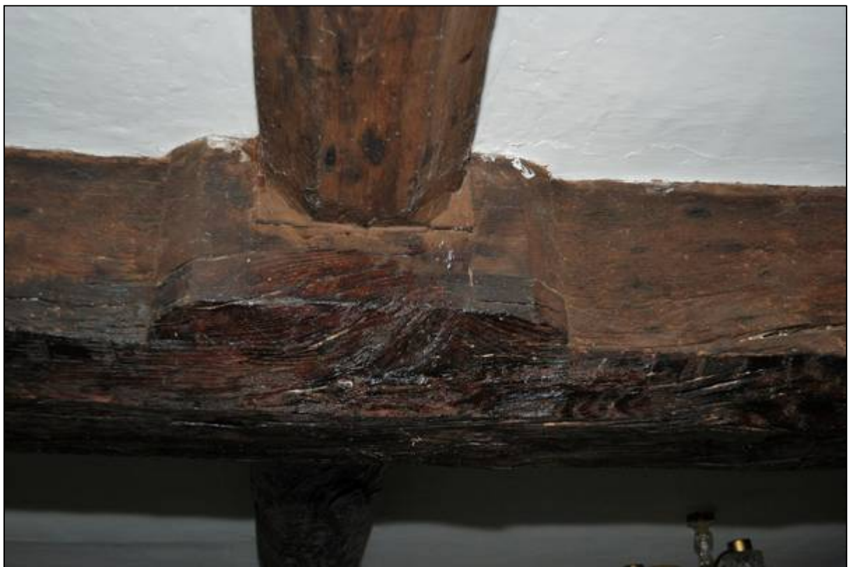
Plate 50: The joint between the northern axial beam and the transverse beam in the parlour.
