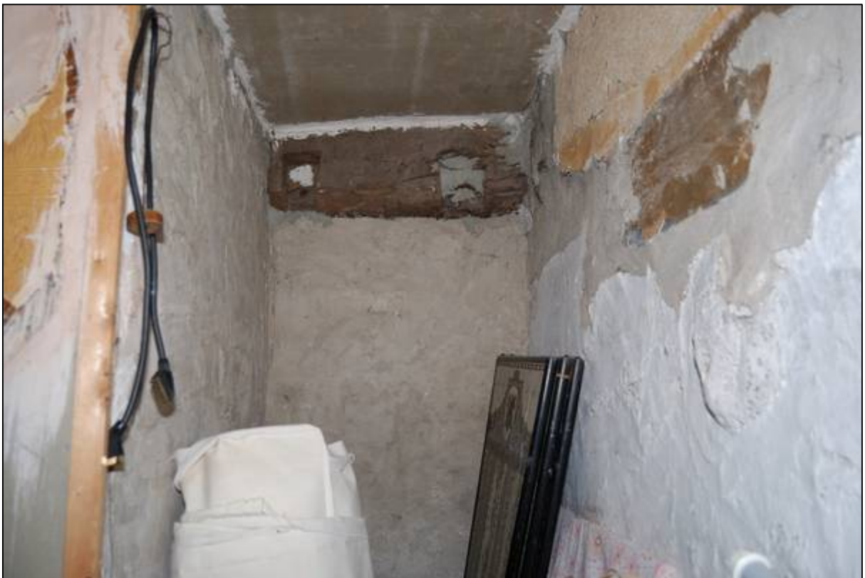
Plate 48: Beam exposed in the below stairs cupboard
