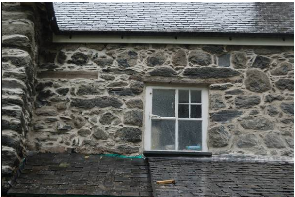
Plate 24: Lintel for the blocked window in the northern face of the “Kitchen Range”
