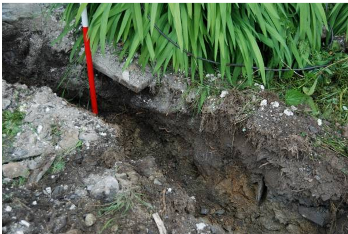
Plate 73: Context 3, foundation trench for the house
