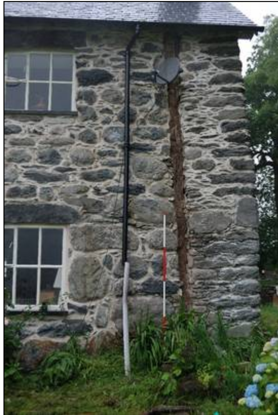
Plate 7: Wooden post exposed by the restoration works
