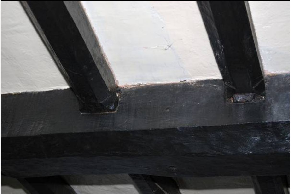
Plate 47: Joists in the hall
