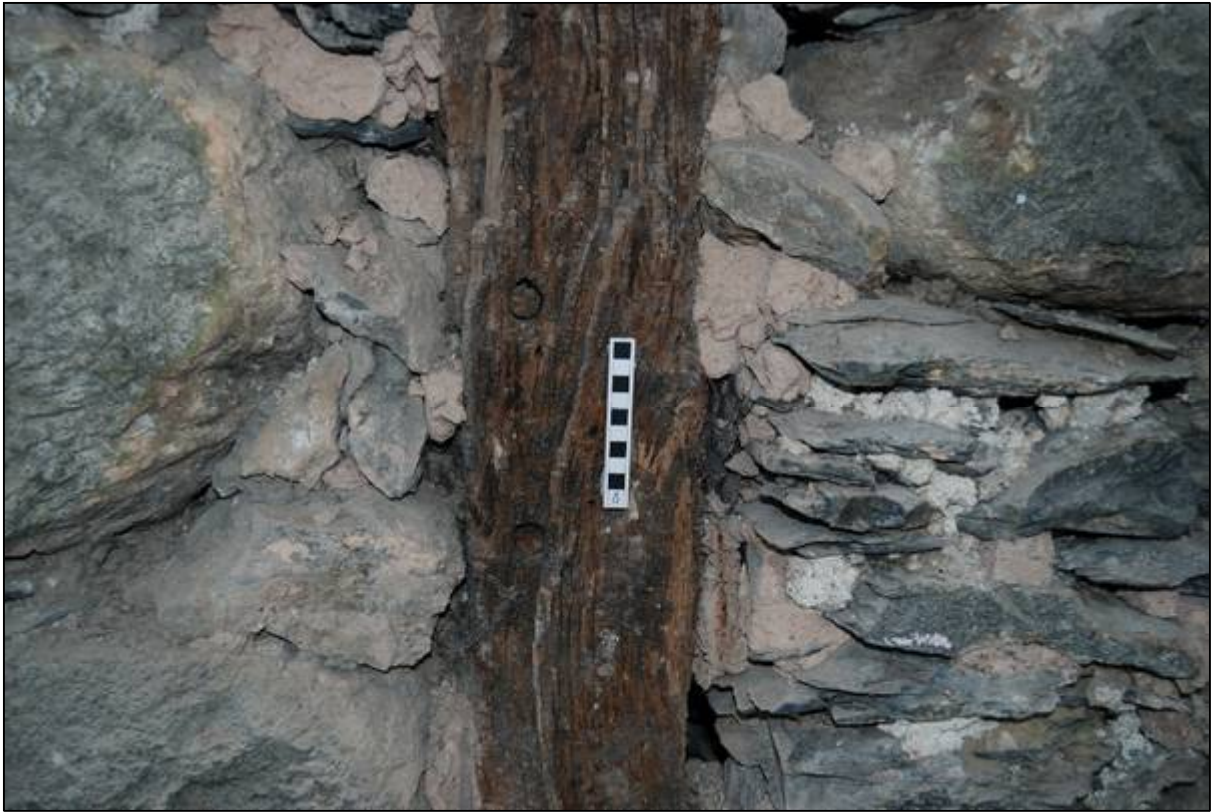
Plate 11: Pegs for a mortice and tenon joint in the external post
