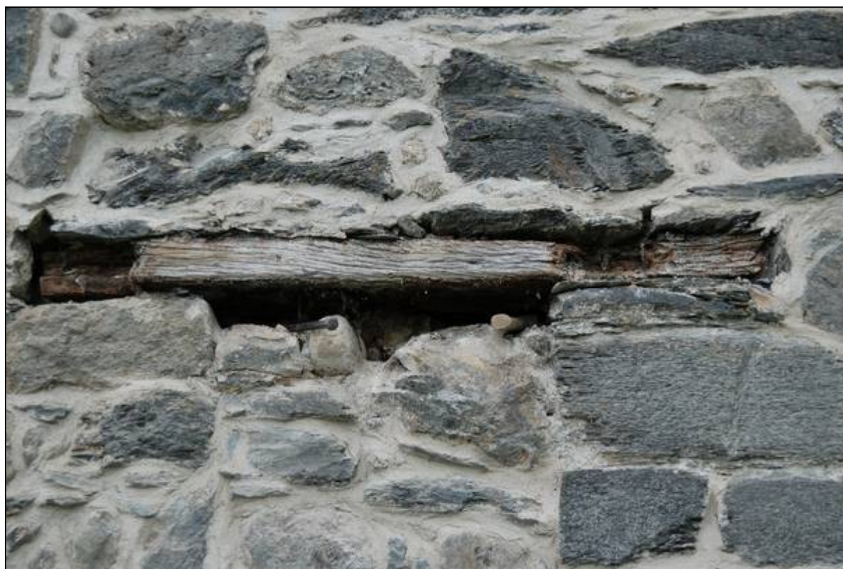
Plate 18: Lintel above the blocked doorway
