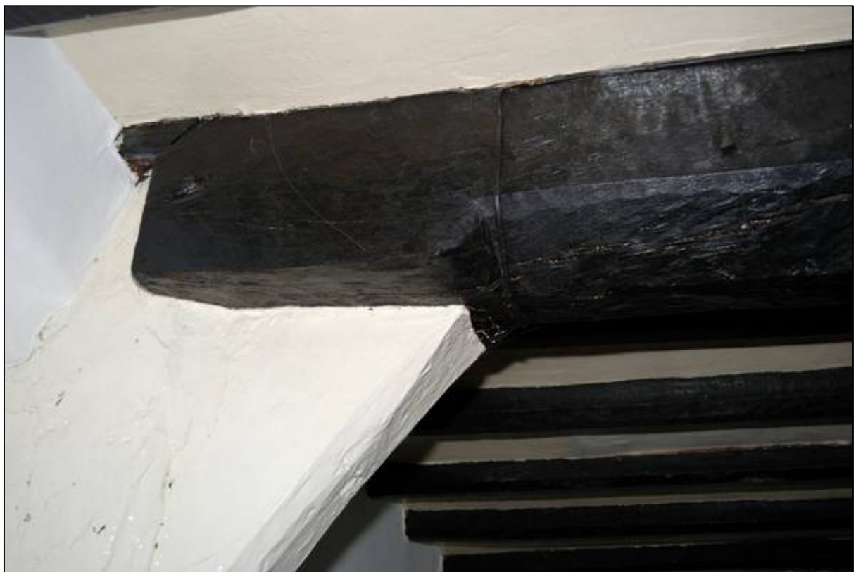
Plate 44: The relationship between the transverse ceiling beam and the post in the hall
