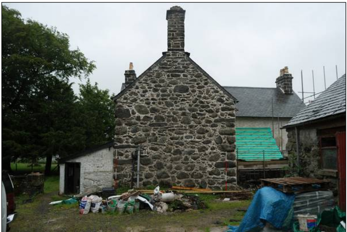
Plate 34: The western elevation
