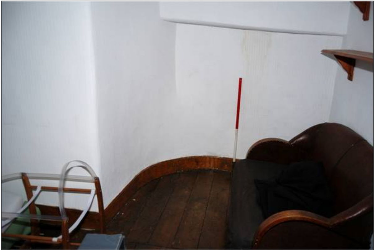
Plate 59: Curved wall in Bedroom 4
