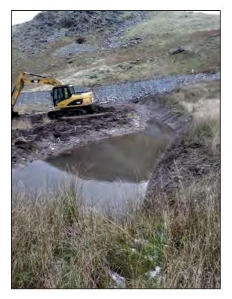
Plate 9: Emergency drain at base of western slopes of Cribau
