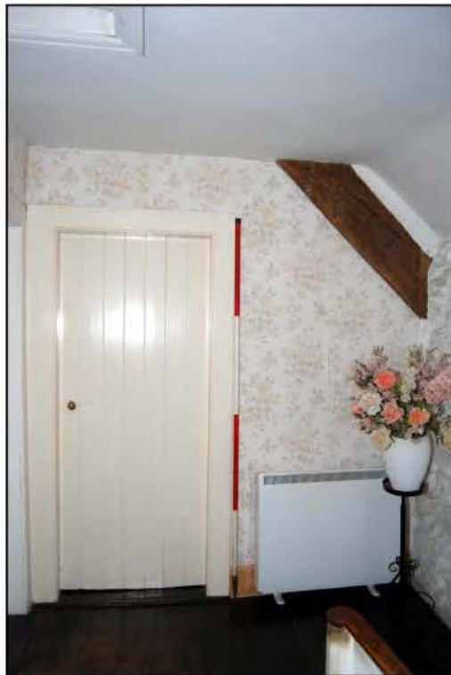
Plate 28: Base of Truss 5, exposed on the landing
