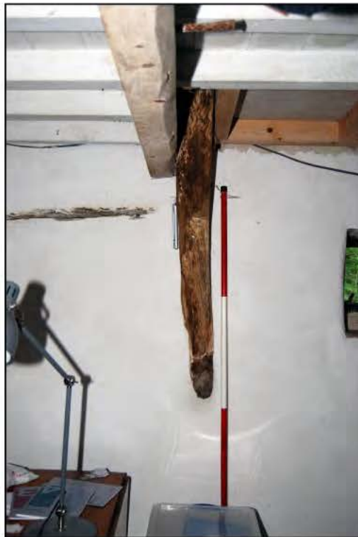
Plate 30: The southern cruck blade in the lower western room
