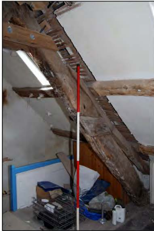
Plate 13: The northern principal rafter of Truss 1
