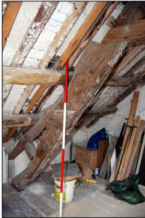
Plate 15: The southern principal rafter of Truss 1
