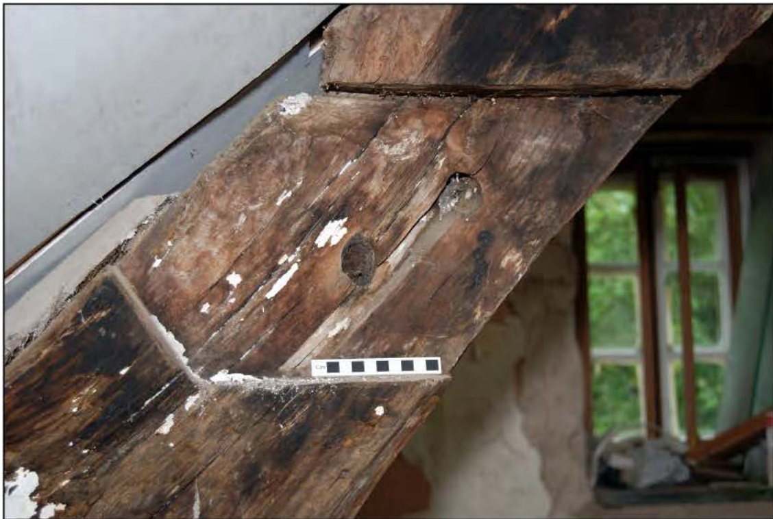
Plate 36: Socket for the collar on the southern blade of Truss 2
