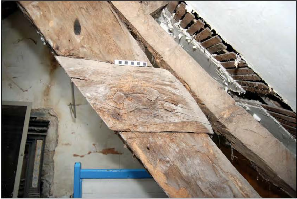
Plate 19: Candle mark on Truss 1
