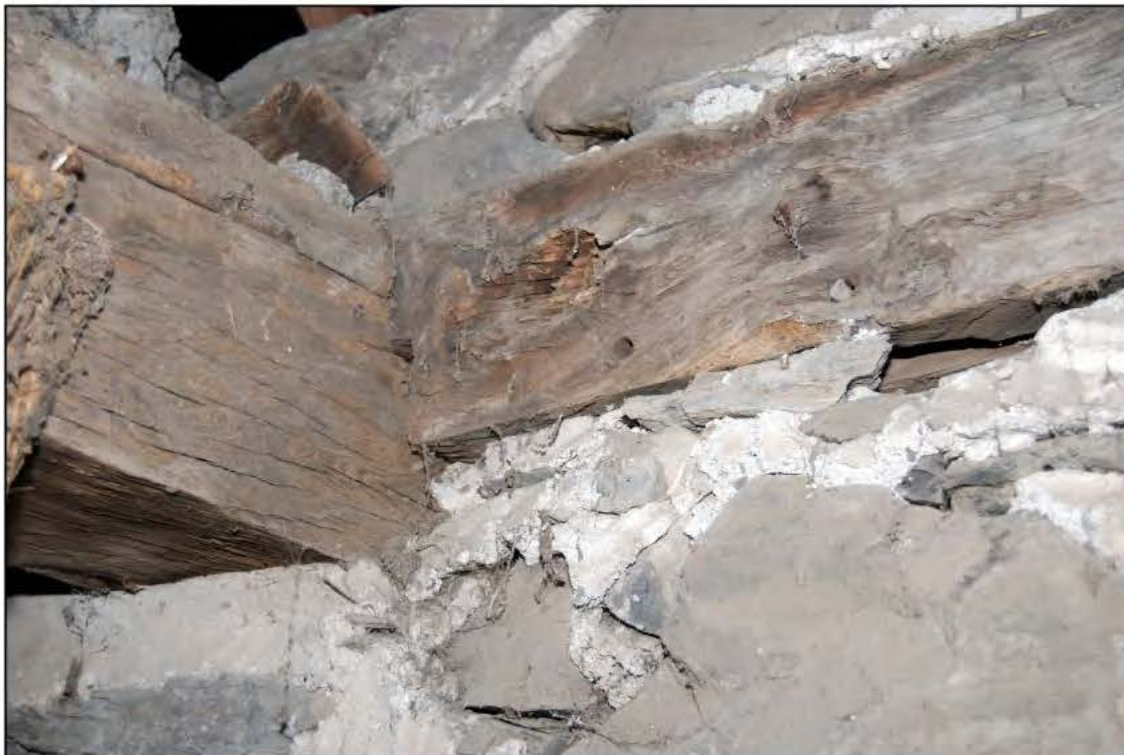
Plate 19: Joint between the rail and the platform
