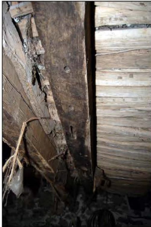
Plate 17: Evidence for the partition below Beam 4
