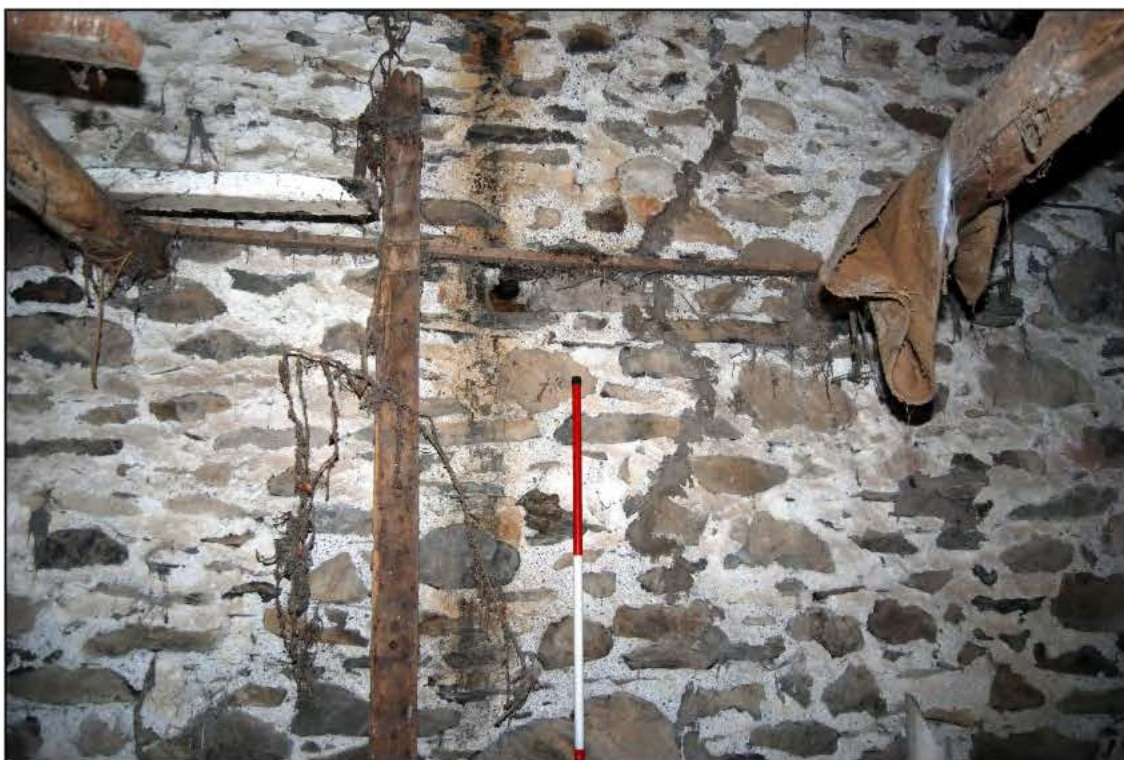
Plate 20: Lateral beams and socket for missing support
