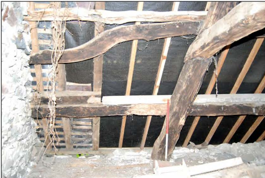
Plate 27: The western end of the northern purlins
