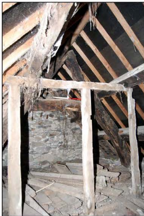
Plate 21: Joints in top of lateral beam
