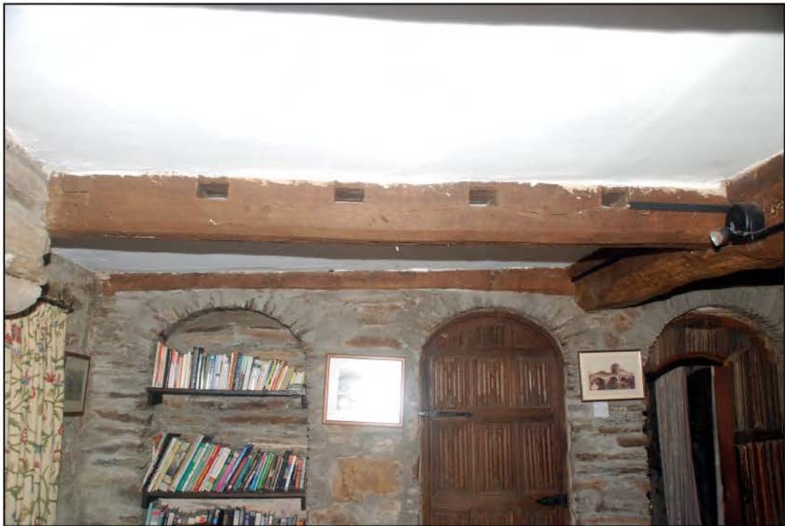
Plate 19: Mortice holes for joists in the parlour
