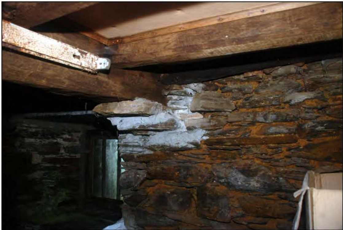
Plate 13: The corbel supporting the transverse beam in the cellar
