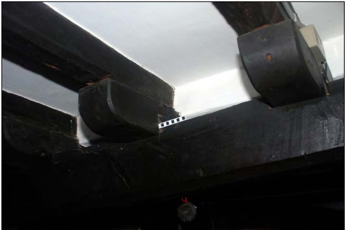
Plate 15: Two level of joists in the hall
