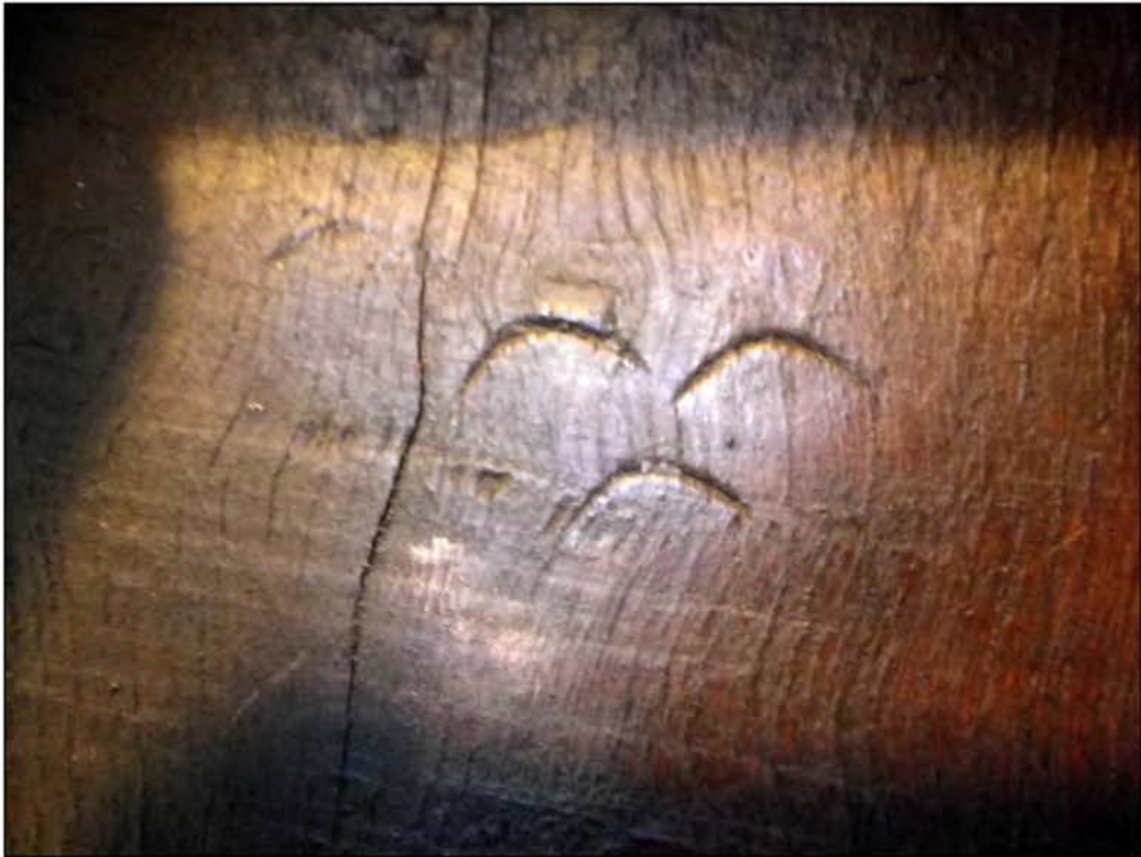
Plate 25: Carpenters marks on the stair partition
