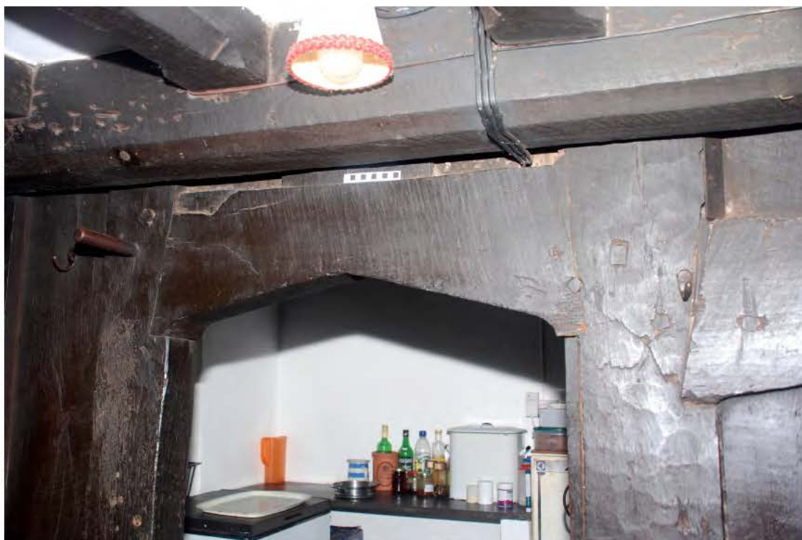
Plate 13: The northern door head
