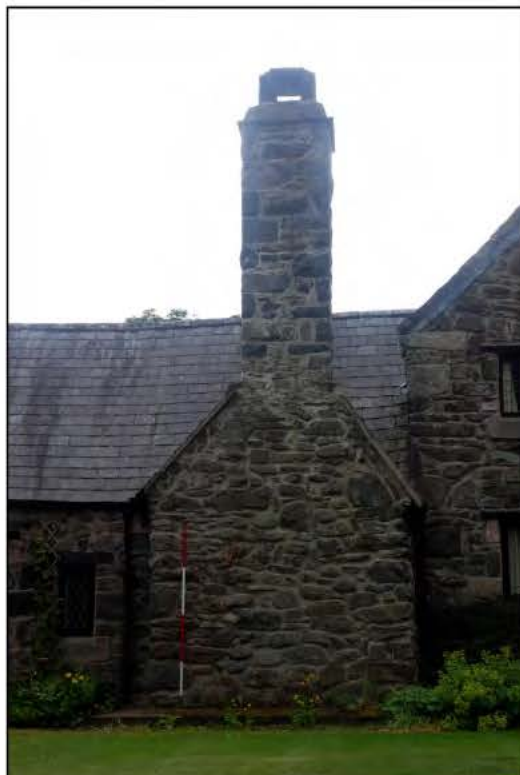
Plate 2: The lateral chimney
