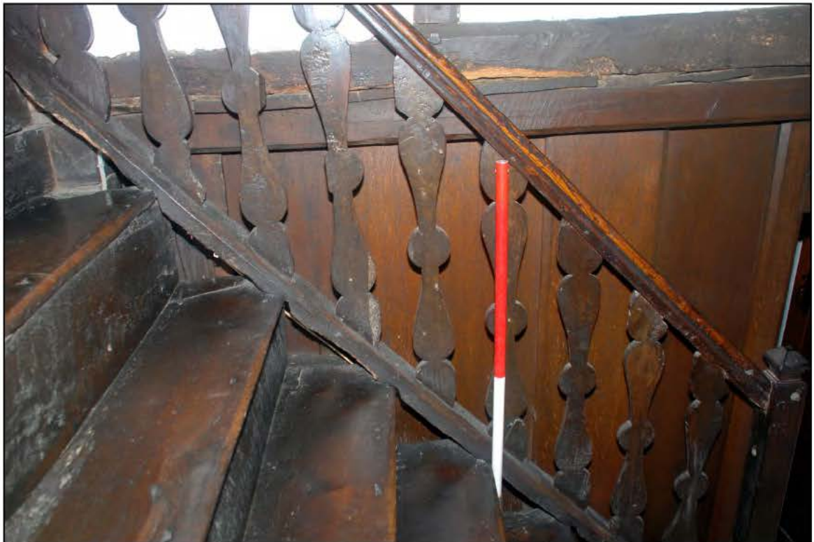
Plate 26: Splat Balusters
