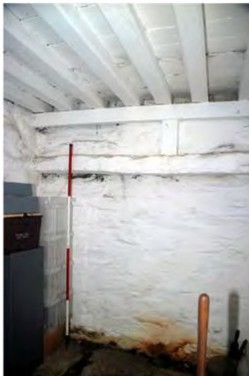
Plate 8: Timber across the northern gable end.
