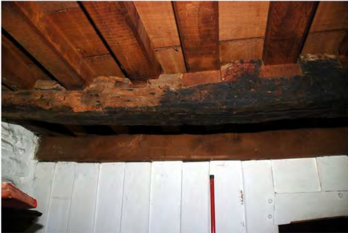
Plate 11: Replacement joists
