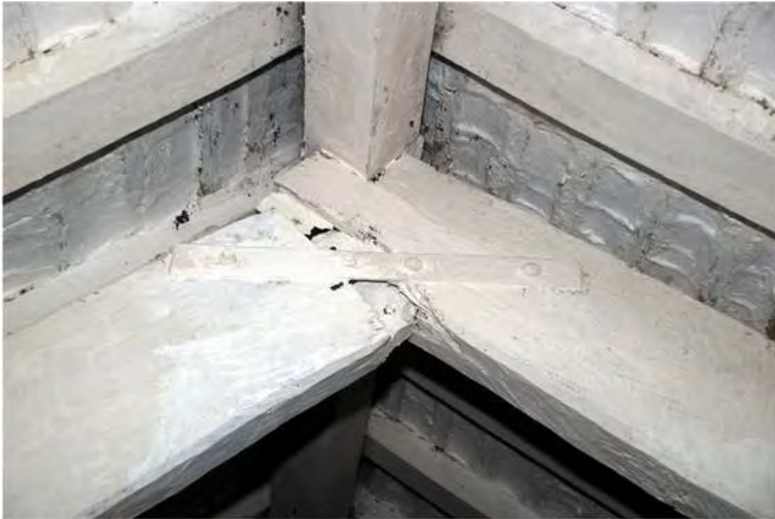
Plate 17: Iron Plate strengthening Truss 1
