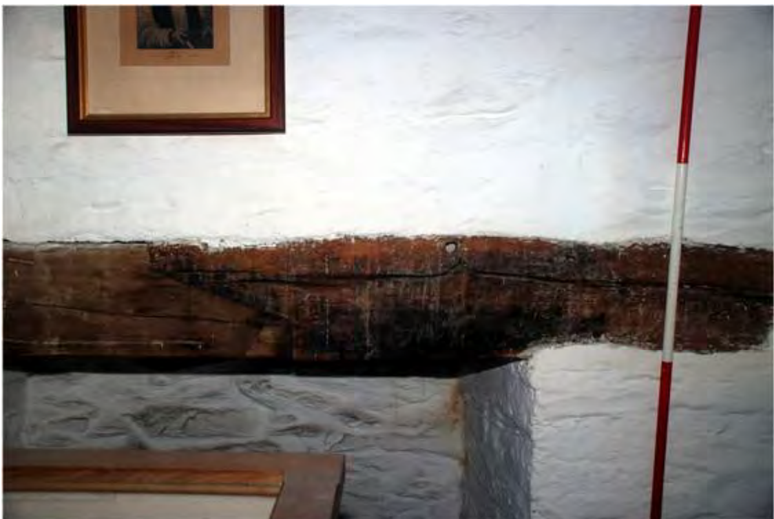
Plate 20: Detail of the repair to the bressumer over the fireplace in the northern gable.
