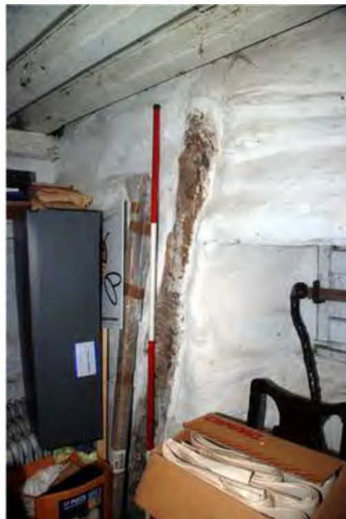
Plate 6: Timber embedded in the wall of the north east ground floor room
