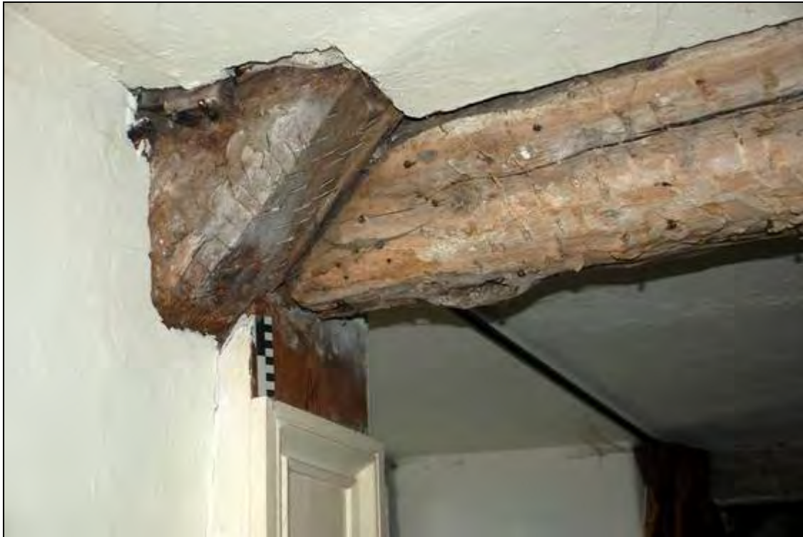
Plate 39: Relationship between the foot of Truss 5 and the tie beam, looking north
