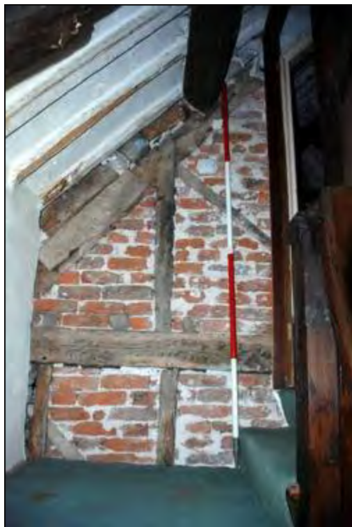
Plate 38: Brick and timber wall in staircase, second floor landing
