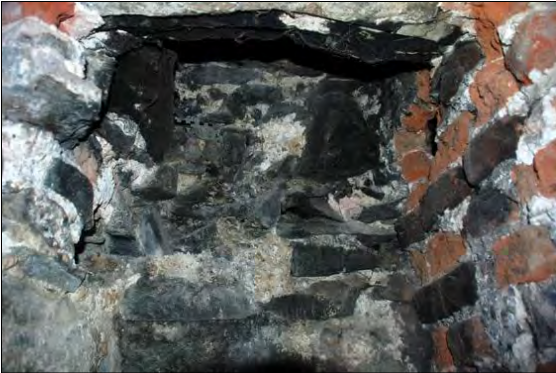
Plate 31: Sooting in stone lined channel on first floor tower room, looking up
