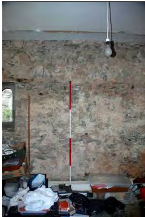
Plate 57: Heightening of the south western wall of the south wing, looking SW
