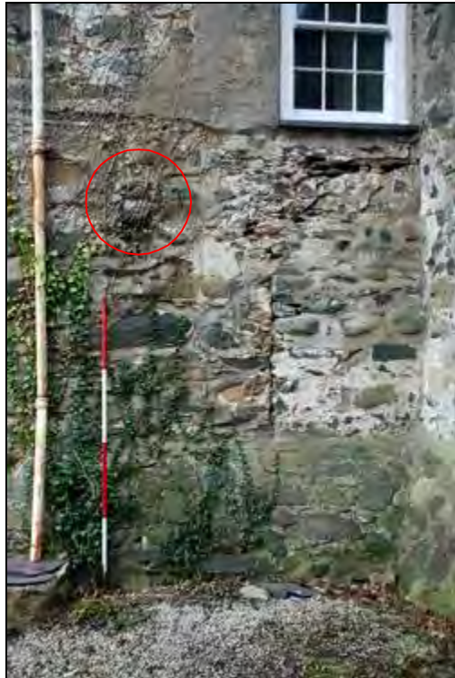
Plate 11: Blocked opening in rear of central range, looking NW (blocked timber socket ringed)
