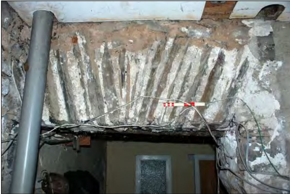
Plate 17: Voussoir head to doorway between north eastern range and north wing
