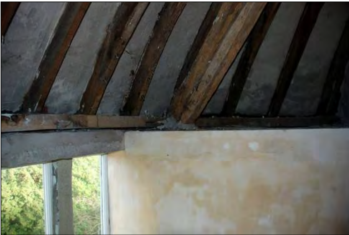
Plate 32: Segmented ring beam supporting the tower roof structure
