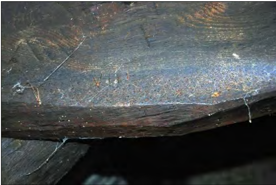
Plate 55: Carpenters marks on Truss 2, looking SW
