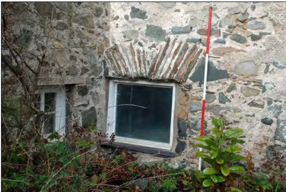
Plate 16: Voussoir head to rear window in the north eastern range, looking west
