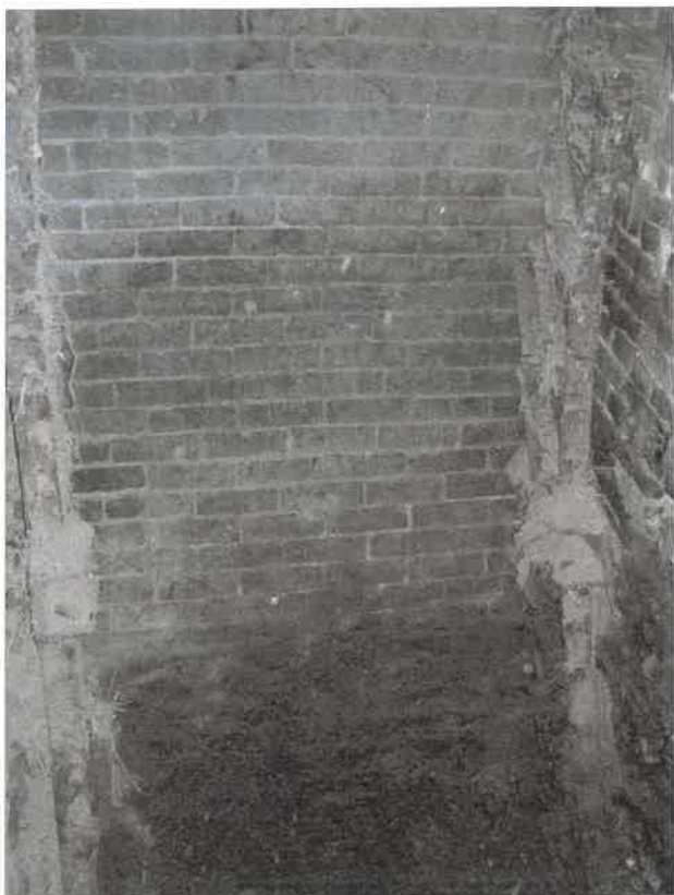
Plate 11: Brick lining at east end of wheel pit
