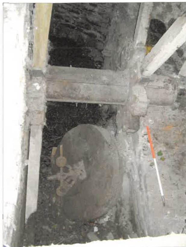
Plate 12: Mill stone lodged in wheel pit, Burr Stone bed stone with governor visible
