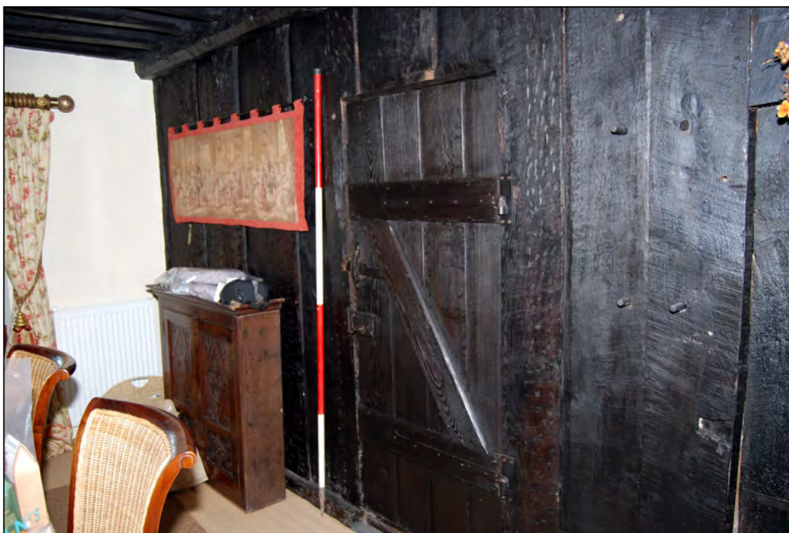
Plate 22: The partition in the parlour, looking SE
