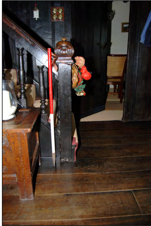
Plate 13: The ground floor section of the staircase
