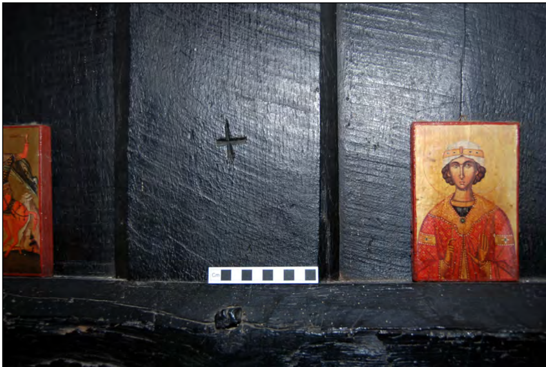
Plate 19: Carpenter's mark on the ground floor partition
