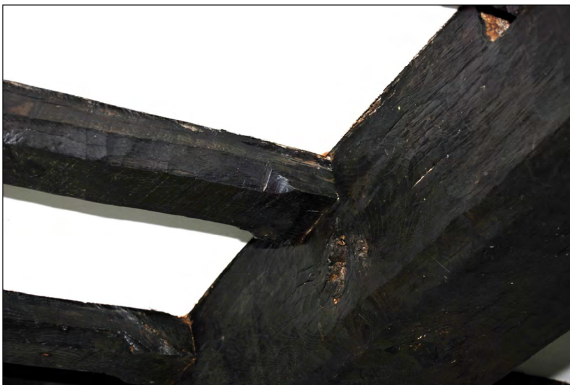
Plate 28: The joists in the bathroom
