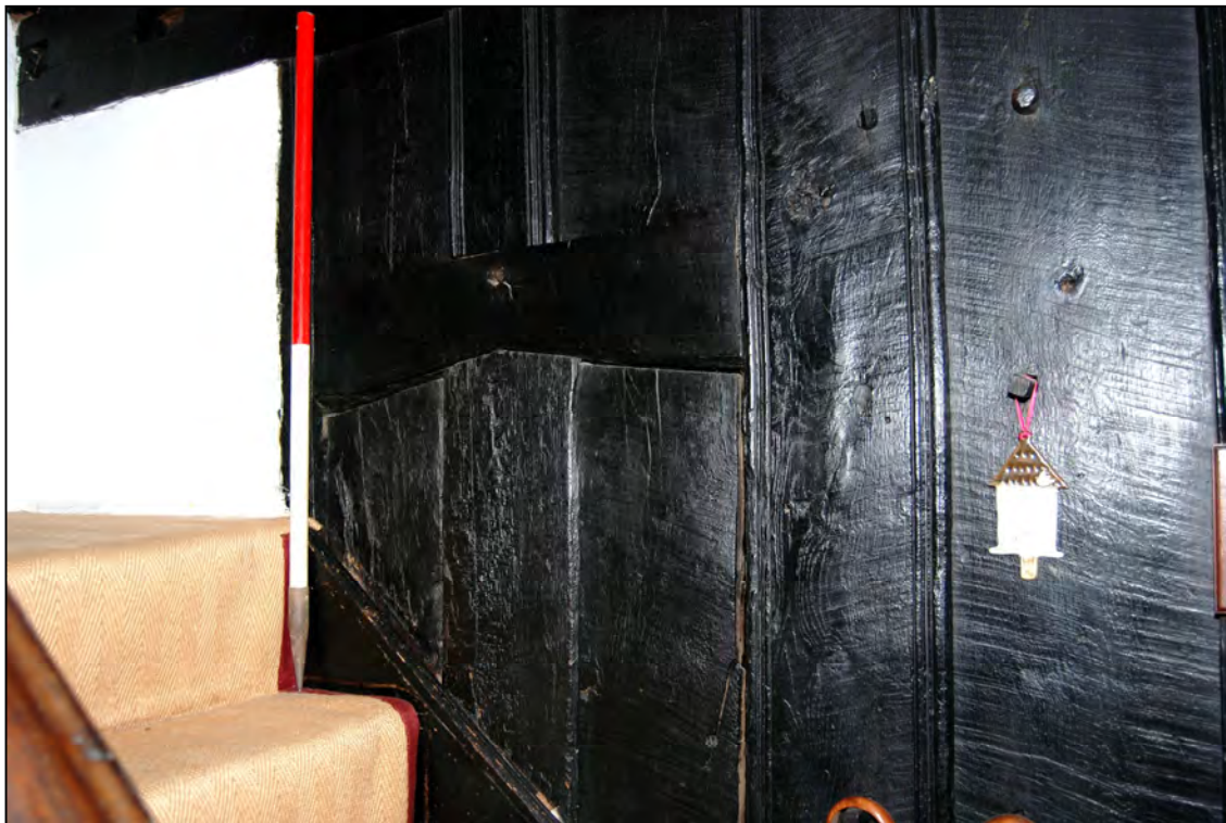
Plate 16: Door head in the partition
