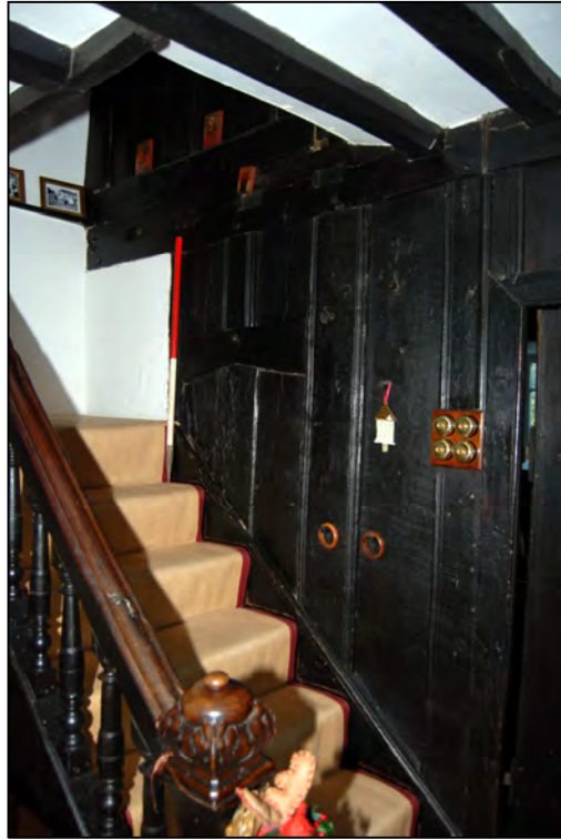
Plate 15: Doorway blocked by the staircase
