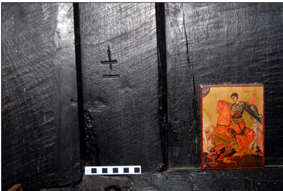
Plate 20: Carpenter's mark on the ground floor partition
