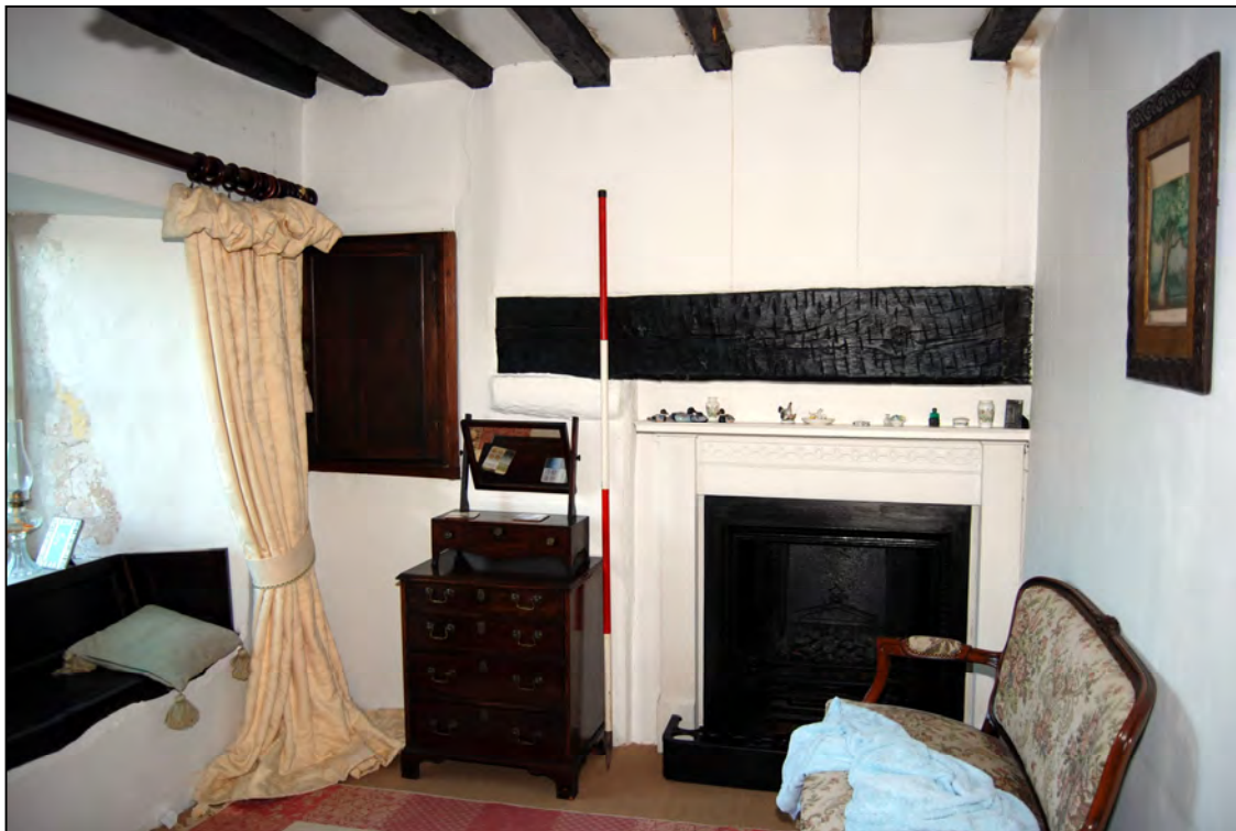
Plate 29: South eastern bedroom
