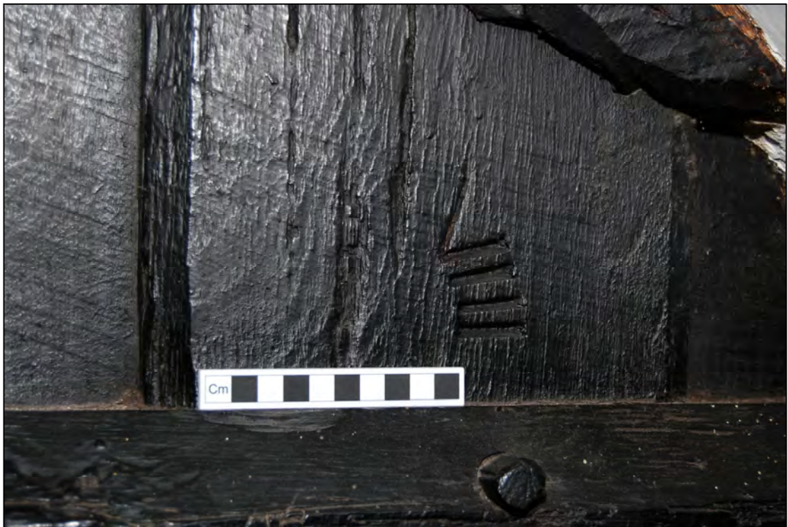
Plate 18: Carpenter's mark on the ground floor partition
