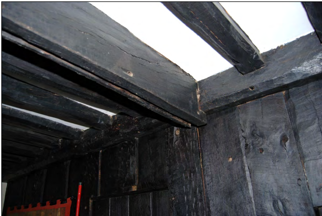
Plate 24: Slot below a joist in the parlour
