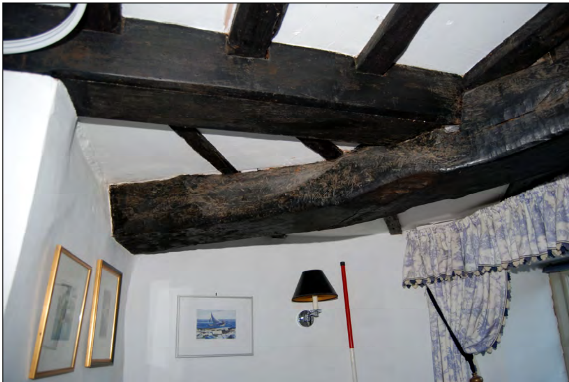
Plate 27: Arrangement of the beams in the bathroom
