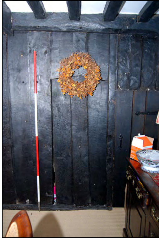
Plate 23: The blocked doorway in the parlour
