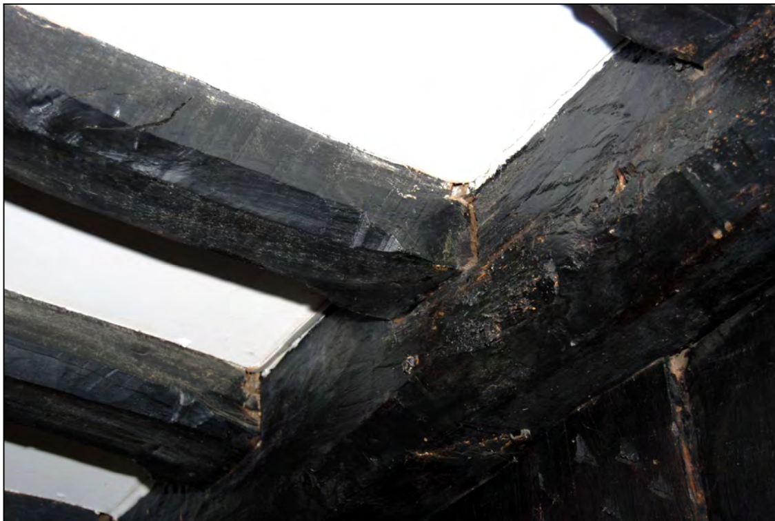
Plate 25: The joists in the parlour
