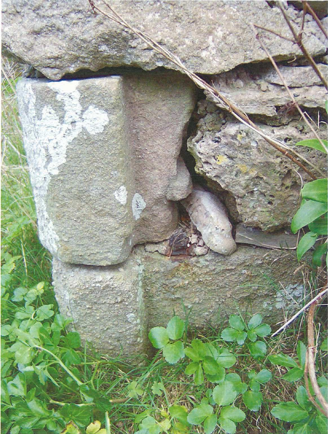
Plate 1: Chamfered jamb in south-west doorway into hall of Block B
