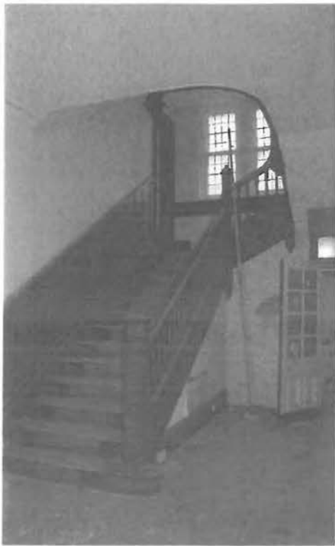
Plate 17: Staircase & hall floored with 4" wide pine boards
