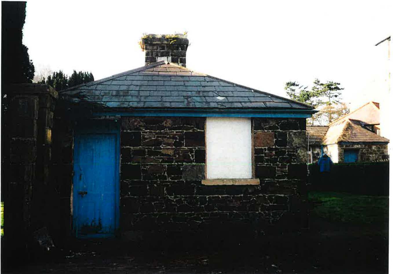
Plate 2 below: Western gatehouse, east elevation; single door with slate threshold & blocked opening with stone sill.
