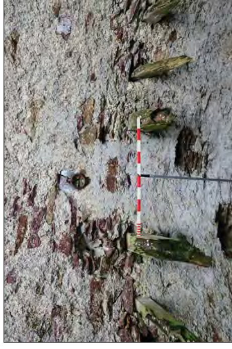
Plate 51. Surviving Joists and Iron Ring. Second Floor Level. Photograph Taken Facing North
