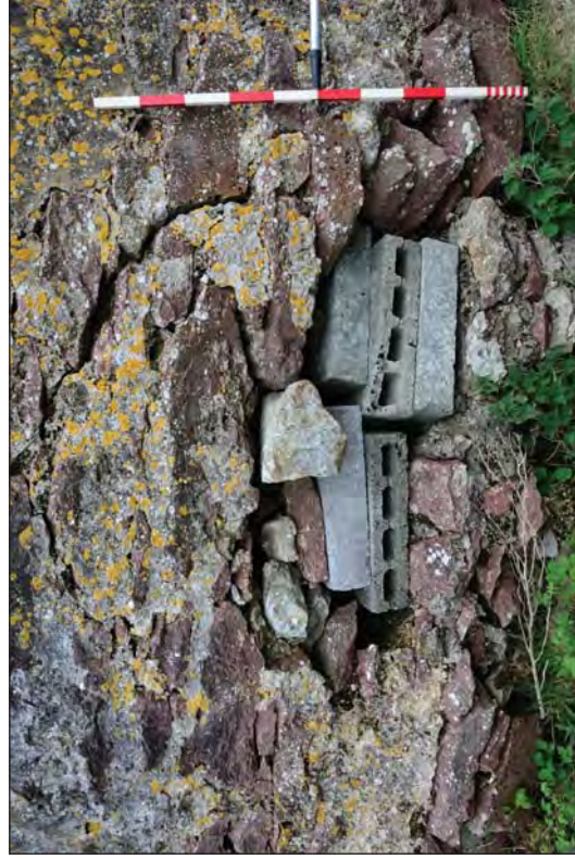
Plate 29. Detailed Shot Showing Lower Blocked Window and Cleat Hole in Eastern Elevation
