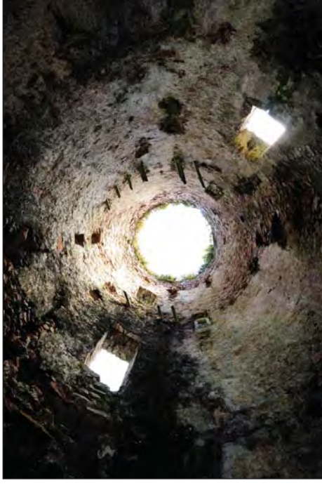
Plate 44. Windmill Interior Showing Surviving Wooden Floor Joists at Second Floor Level
