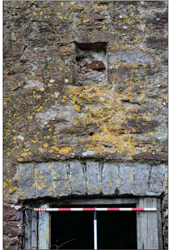
Plate 25. South-eastern Doorway Showing Limestone Detailing
