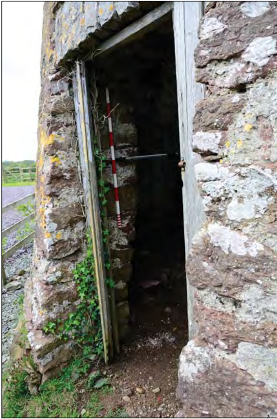
Plate 24. South-eastern Doorway Showing Wall Thickness
