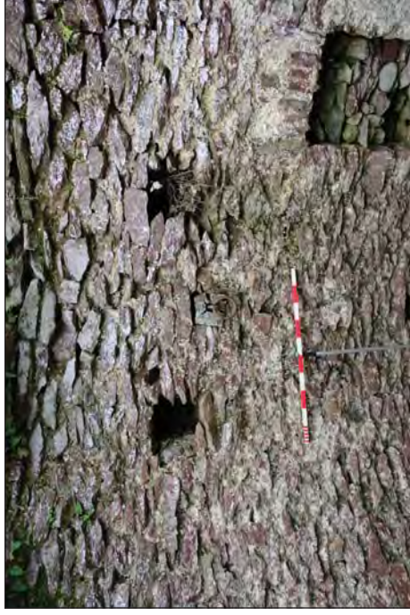
Plate 45. Joist Holes for Third Floor Level. This Level Would Have Been Inside the Windmill Cap
