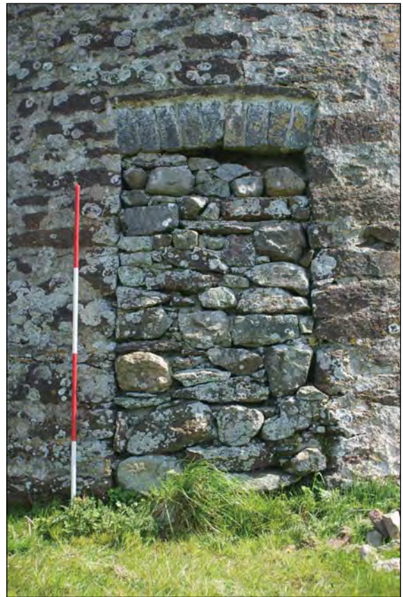
Plate 17. Blocked Doorway in North-western Elevation
