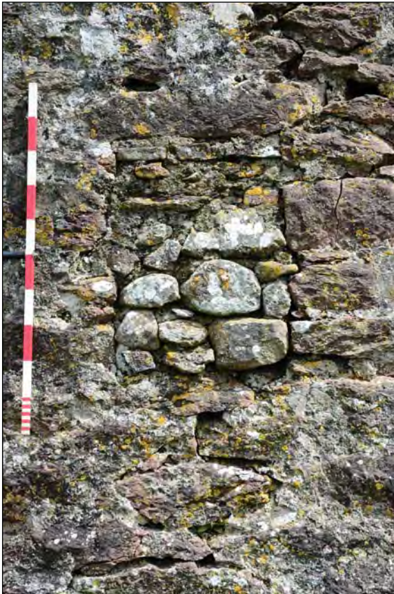
Plate 26. Blocked Window Lower Level Western Elevation
