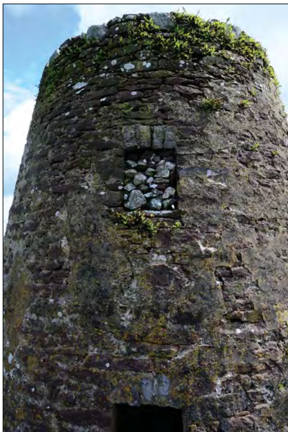
Plate 32. Blocked Second Floor Window in Western Elevation
