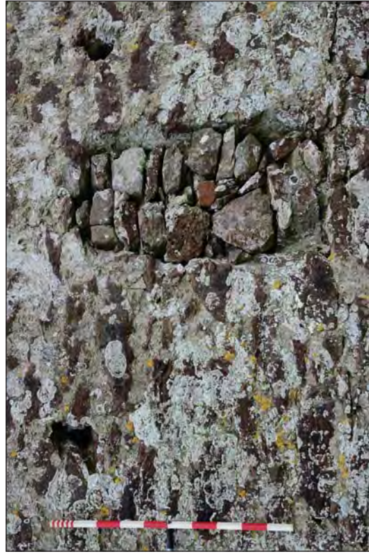
Plate 28. Detailed Shot Showing Location Of Cleat Holes on the Southern Elevation of the Tower
