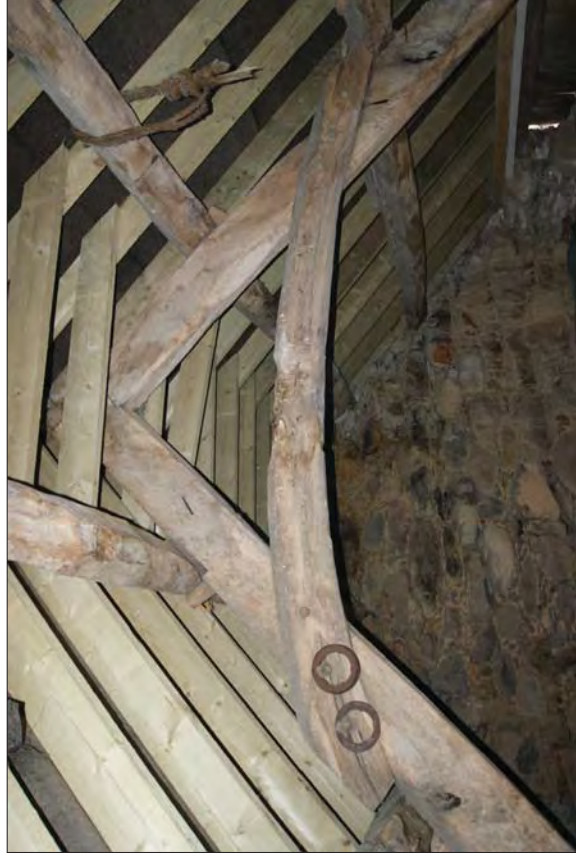
Plate 30. Roof Detail Showing Original Wooden Frame and Modern Replacement Roof and Rafters
