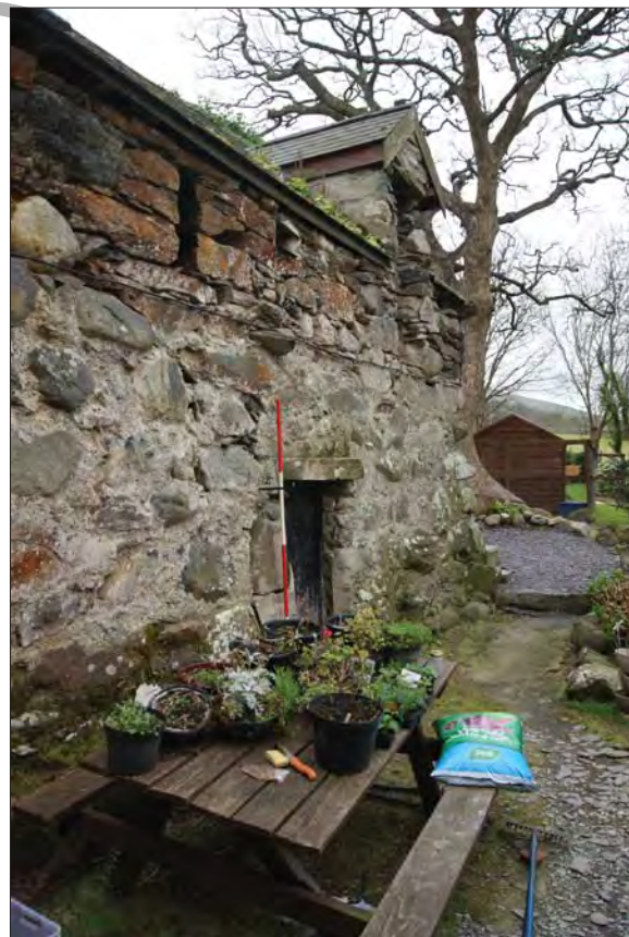
Plate 24. Rear Elevation Detailing Large Boulders Projecting at Ground Floor Level
