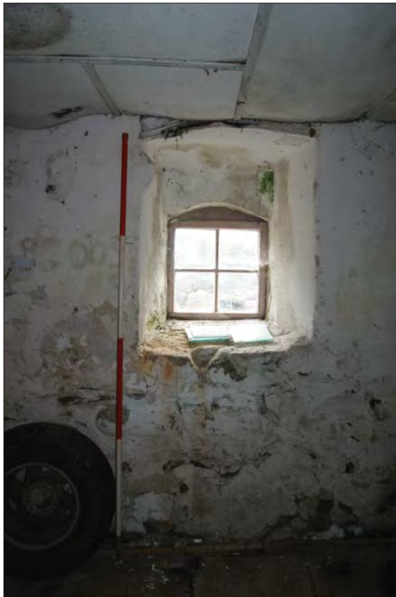
Plate 45. Ground Floor Window in Front Elevation. Later Blocking Evident
