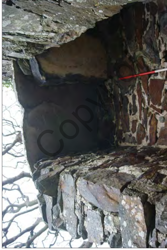
Plate 25. Large Slabs Roofing External Stairway
