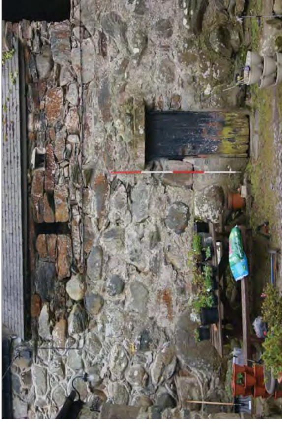
Plate 18. Rear Elevation Showing Later Addition of First Floor
