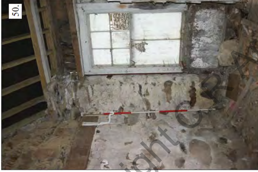
Plate 49. Ground Floor Rear Wall Following Removal of Wooden Panelling Plate 50. Ground Floor Front Wall Following Removal of Butcher's Shop Fittings Plate 51. Ground Floor Following Removal of Floor Plate 52. Ground Floor Following Removal of Floor (Taken from First Floor Level)
