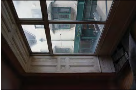
Plate 59. Surviving Panelling Around Modern Window
