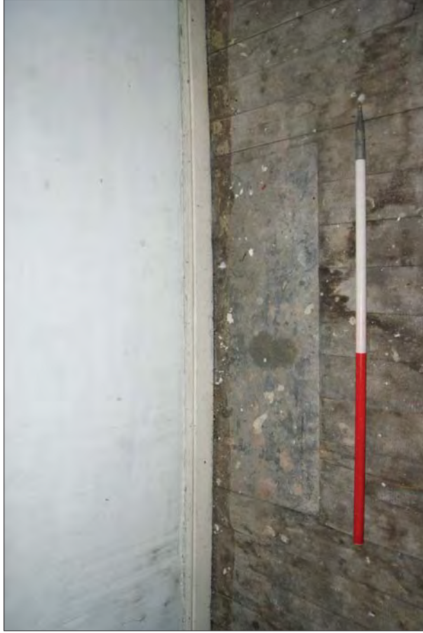
Plate 85. Slate Hearth Stone in Attic Room 2
