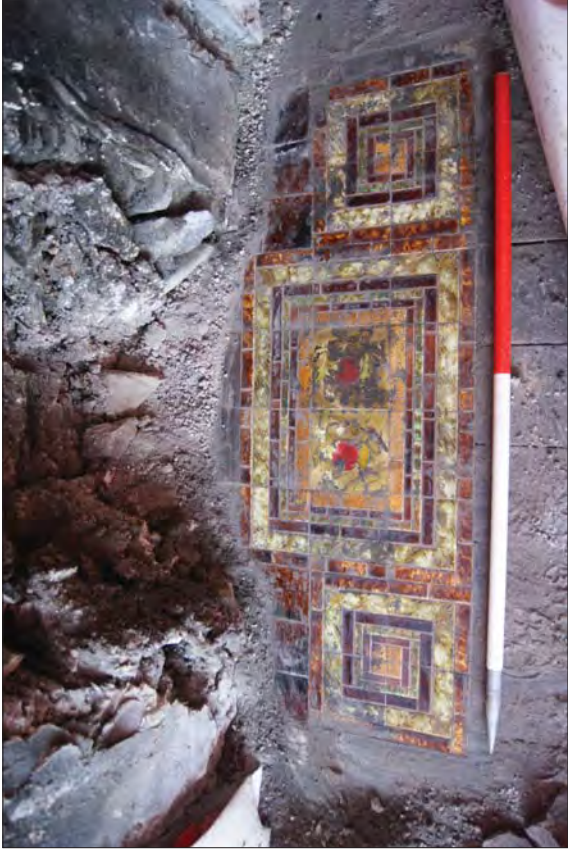
Plate 63. Surviving Victorian Ceramic Tiles in Hearth of Destroyed Fireplace
