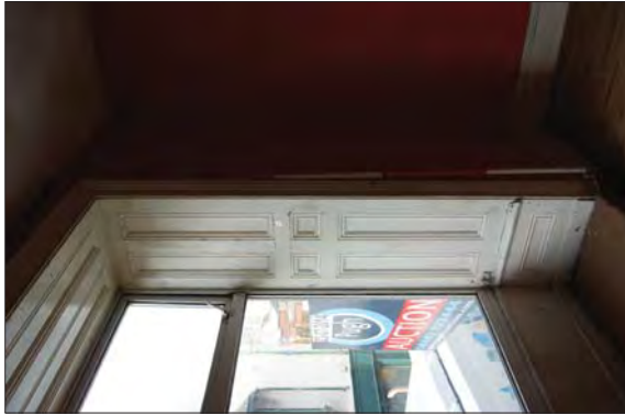
Plate 59. Surviving Panelling Around Modern Window
