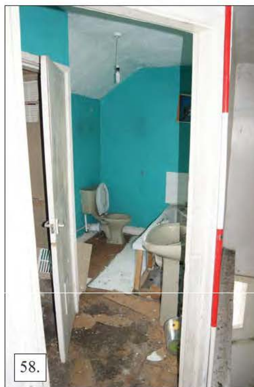
Plate 58. Bathroom at Rear of Unsafe to Enter Due to Rotten Floor
