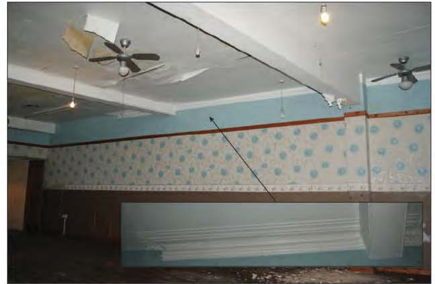
Plate 43 (And Inset). First Floor Shop Space Showing Surviving Plaster Cornice Detail
