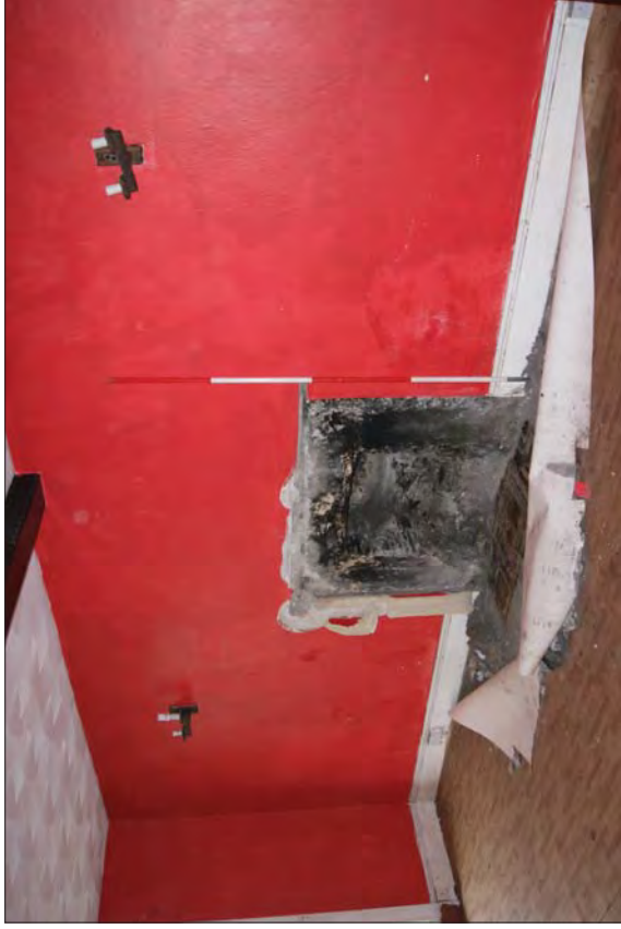
Plate 61. Surviving Panelling Around Modern Window Originally Housed a Bay Window Which has been Removed
