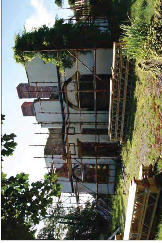
Plate 6. Crenellations of Previous Boundary Wall Later Integrated into Rear Extension Wing
