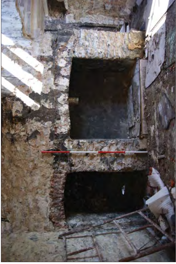
Plate 54. Fireplace/Oven in Kitchen Showing Flue in Doorway
