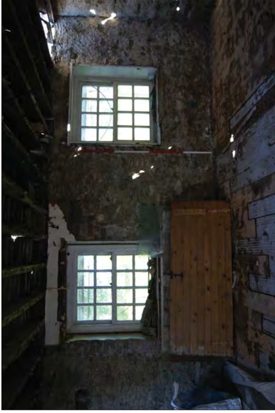
Plate 72. Western Extension Showing Modern Replacement Windows in Original Openings
