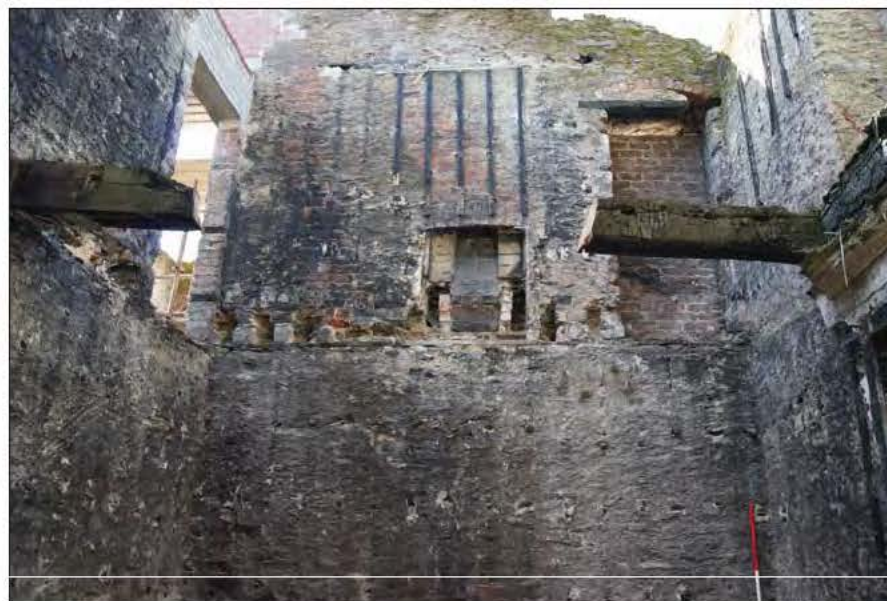
Plate 43. First Floor Opening for Fireplace and Closet Which Appears To be Bricked Doorway. Note Timber Studs for Plasterwork
