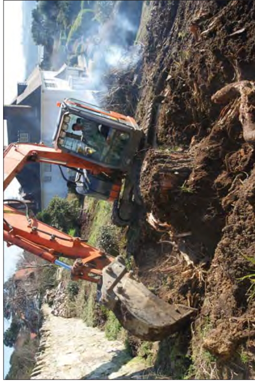
Plate 5. Machine Removal of Tree Stumps
