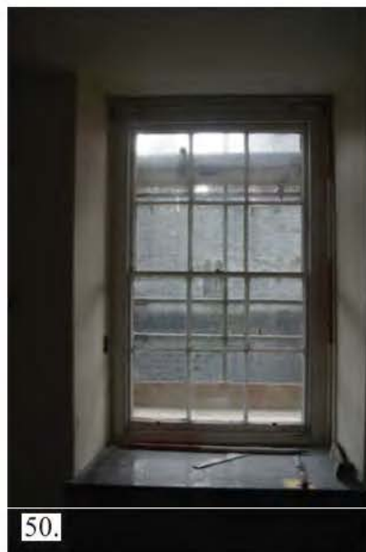
Plate 49 - 50. First Floor Room 16 Showing Enlarged Opening and Sash Window
