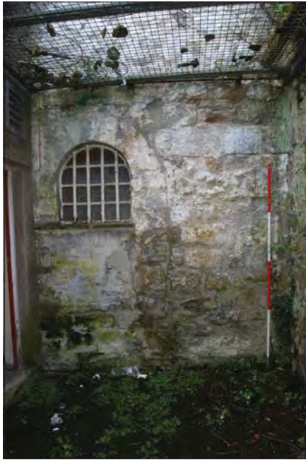
Plate 7. Rear Elevation Showing Blocked Doorway & Window of Room 6
