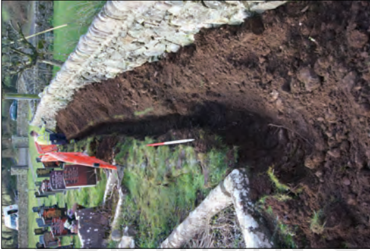
Plate 1. Cable Trench Running Alongside Churchyard Wall
