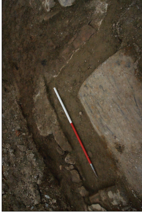
Plate 6. Surviving Cellar Wall Constructed Using Red Sandstone
