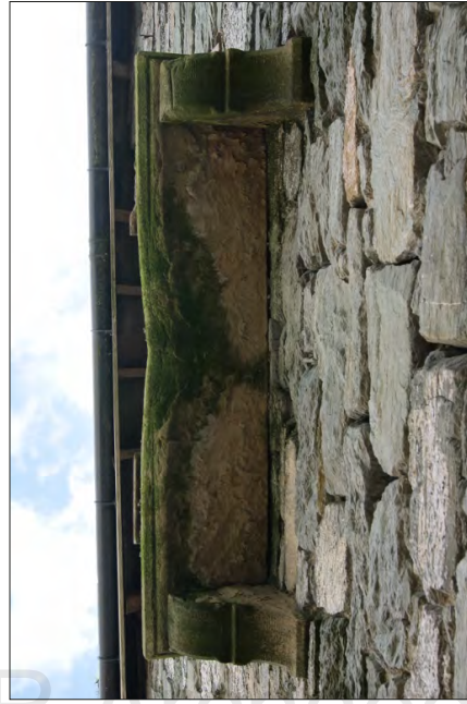
Plate 27. Window Sill Detail - North Facing Elevation
