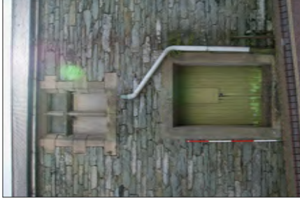
Plate 25. Blocked Window in North Facing Elevation
