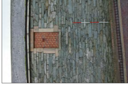
Plate 25. Blocked Window in North Facing Elevation
