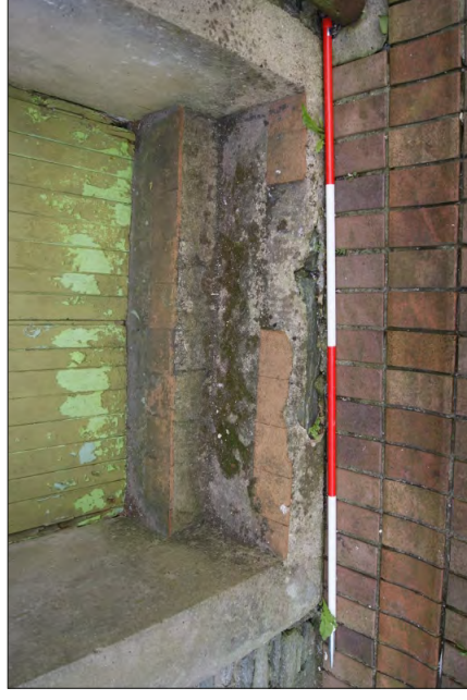
Plate 28. Lower Doorway in North Facing Elevation. Ceramic Tiled Steps
