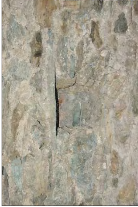
Plate 42. Detailed Shot of Recess Possibly Original Location of Floor Joist
