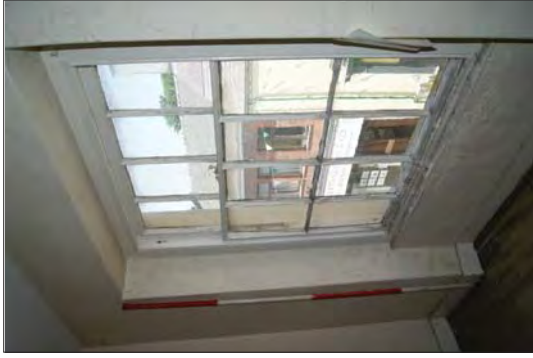
Plate 46. Second Floor Room 8 Four Over Eight Sash Window
