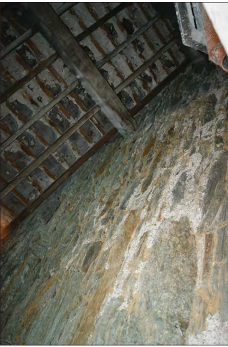
Plate 57. 11 Stanley Street Attic Showing Building Scar Possibly the Remains of an Earlier, Lower Gable Wall Which Was Incorporated into Building
