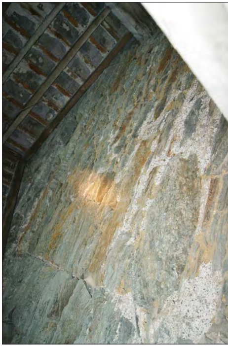
Plate 58. 11 Stanley Street Attic Showing Building Scar Possibly the Remains of an Earlier, Lower Gable Wall Which Was Incorporated into Building
