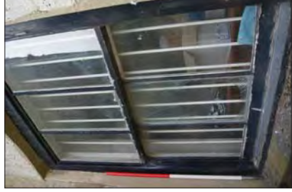
Plate 49. Three Over Three Horned Sash Window Room 9
