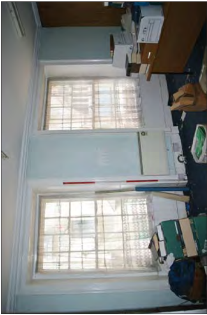
Plate 33. 11 Stanley Street First Floor Room 5 Eight Over Eight Original Georgian Sash Windows
