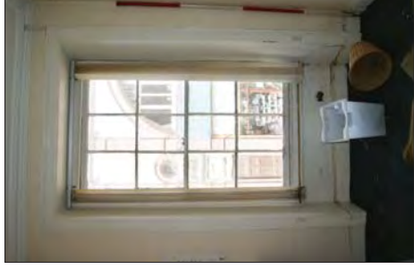
Plate 77. Six Over Six Sash Window Room 4
