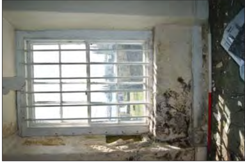
Plate 98. Room 6 Original Eight Over Eight Sash Window
