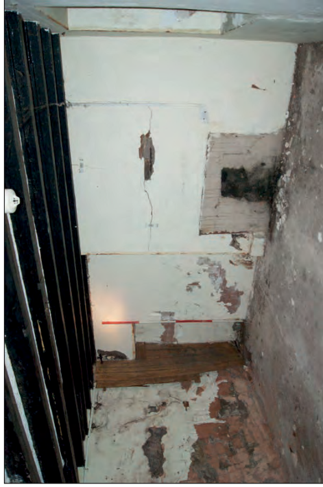
Plate 63. Basement Level Room 13. Note Blocked Doorway in Corner and Blocked Fireplace
