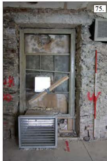
Plates 70 - 76. First Floor Level. Detailed Photographs of Blocked Sash Window in Rear Elevation
