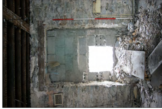
Plate 60. Second Floor Level. Blocked Opening in East Facing Elevation
