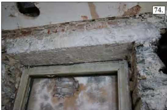
Plates 70 - 76. First Floor Level. Detailed Photographs of Blocked Sash Window in Rear Elevation
