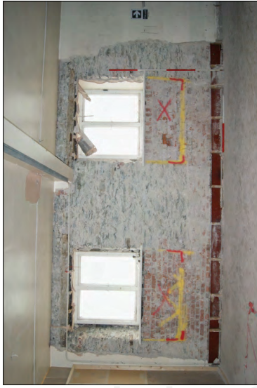
Plate 62. First Floor Level. Blocked Window Details in Front Elevation
