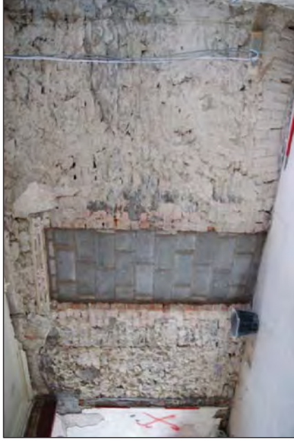
Plate 115. Second Floor Following Stripping Out of Building Showing Concealed Openings
