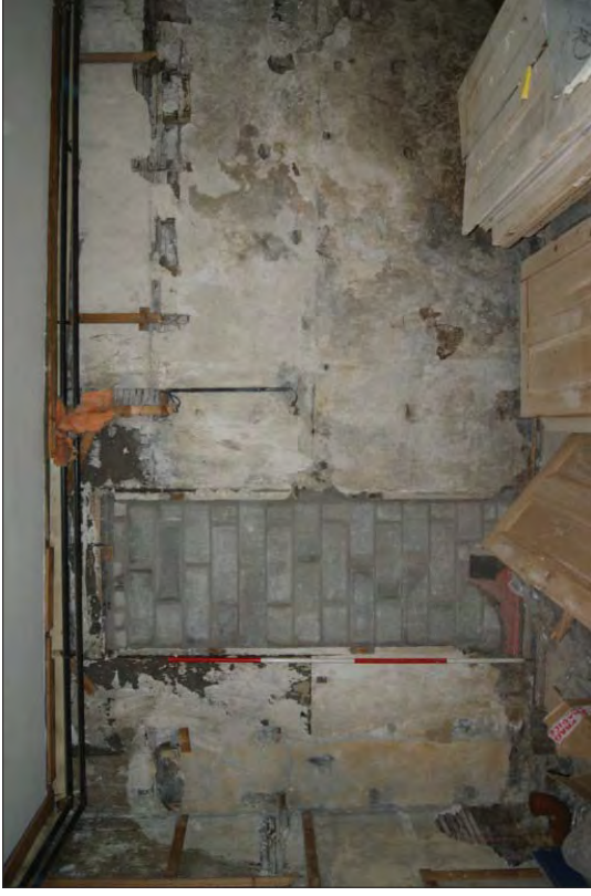
Plate 94. Element 4a Manager's Office Ground Floor Level. Door Re-blocked as Leads to Outside
