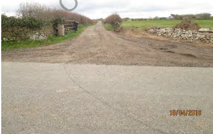
The Access from the public road, in course of splay and visibility improvement
