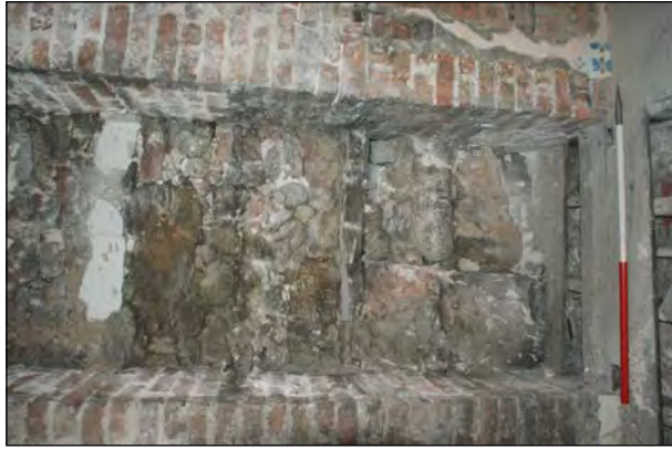
Plate 51. Room 6 First Floor. Gable Wall Showing Partition With Room 5 and Edge Of Fireplace
