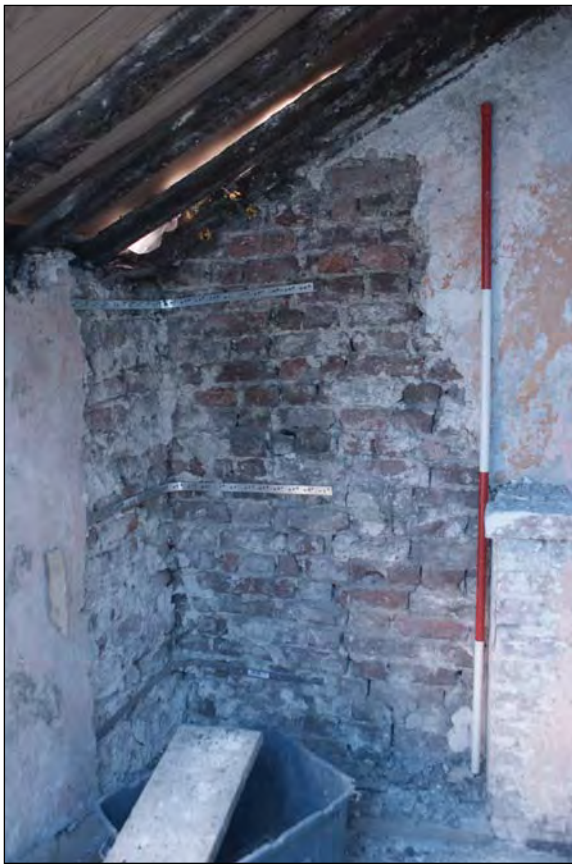
Plate 23. Room 2 Later Brick Facade. The Facade Has Not Been Keyed into the Gable Wall and is Causing Structural Problems
