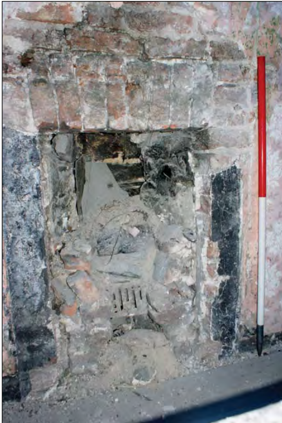
Plate 23. Room 2 Later Brick Facade. The Facade Has Not Been Keyed into the Gable Wall and is Causing Structural Problems
