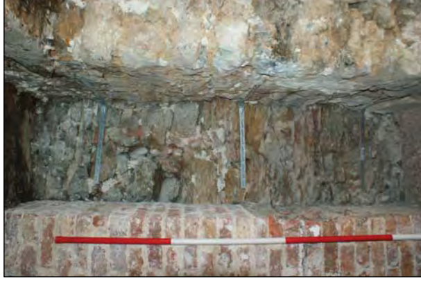
Plate 53. Room 6 First Floor. Gable Wall Showing Join With Rear Wall and Edge Of Fireplace
