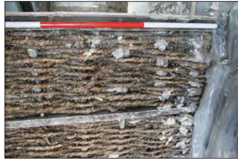
Plate 50. Room 5 First Floor. Rope and Plaster Partition Detailed Shot
