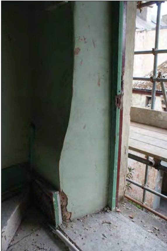
Plate 36. Wall Thickness on Second Floor Stairway Landing
