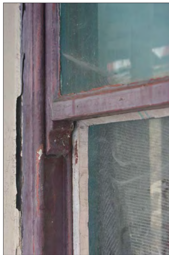
Plate 8. 21 High Street Front Elevation Detailing Left Hand Ground Floor Window Horn
