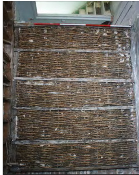
Plate 46. Room 5 First Floor. Rope and Plaster Partition Detailed Shot of Four Panels
