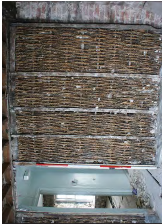
Plate 45. Room 5 First Floor. Rope and Plaster Partition to the Right Hand Side of Door
