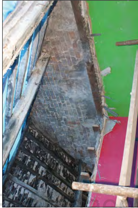
Plate 13. Roof Space Above Room 1. Divides Level in Half. Constructed of Twisted Rope and Plaster. Shows Attic Space
