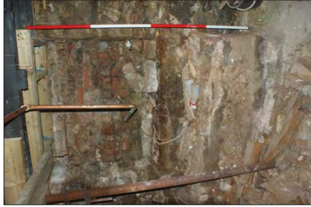
Plate 81. Room 9 Cellar. Steps and Blocking Directly Below the Right Hand Window
