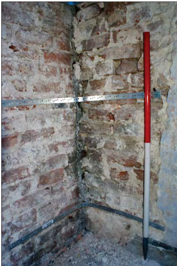
Plate 19. Room 1 Later Brick Facade. The Facade Has Not Been Keyed into the Gable Wall and is Causing Structural Problems
