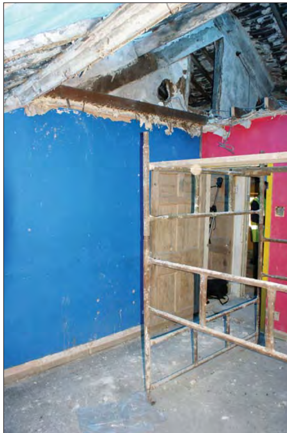
Plate 20. Room 1 General Shot Showing Doorway and Rope and Plaster Room Division
