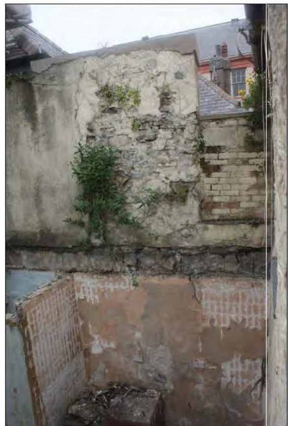
Plate 91. Dividing Wall Showing Blocking Episode
