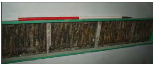
Plate 65. Rope and Plaster Preserved Behind Glass on First Floor Landing
