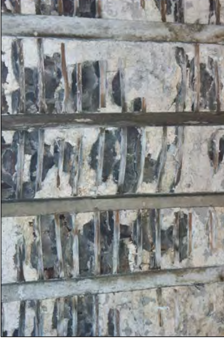
Plate 15. Detailed Shot of Slate Roof Above Room 4. Note the Small Size and Irregular Shape Of the Tiles Used. View From Room 1
