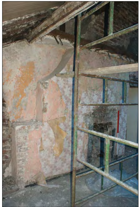
Plate 24. Room 2 Large Brick Chimney Breast. Also Spans Room 3
