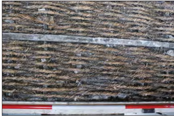
Plate 47. Room 5 First Floor. Rope and Plaster Partition Detailed Shot
