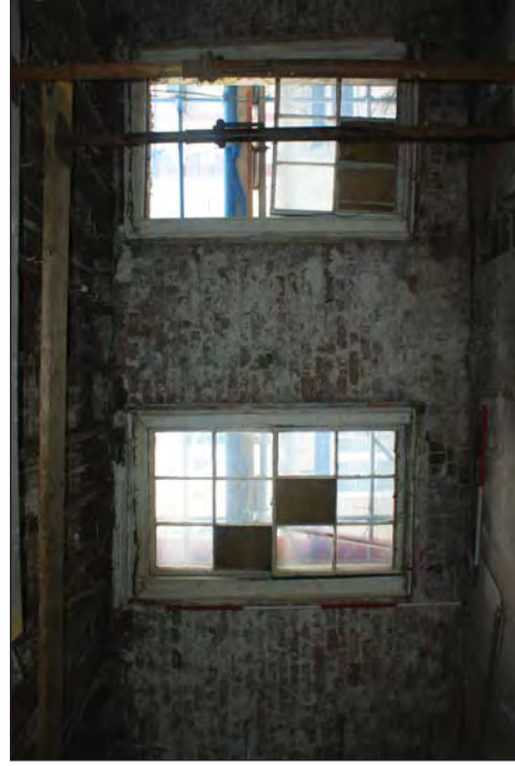
Plate 41. Room 5 First Floor. Sash Windows Facing The Street. Note the Facia Brickwork Below the Windows
