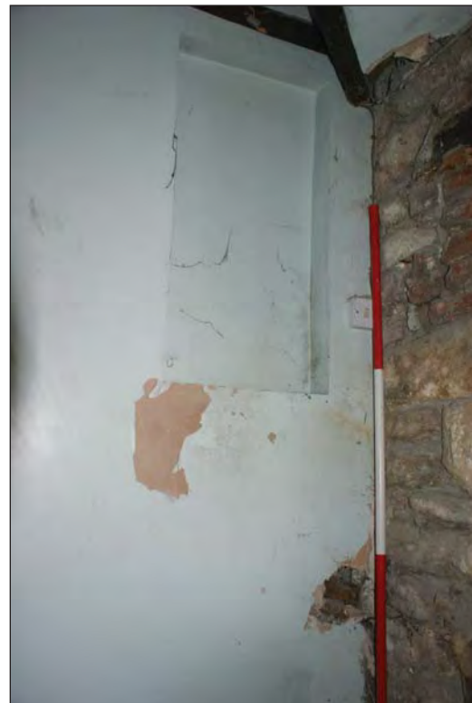
Plate 61. Landing on Stairs First Floor. Blocking of Window/Recess
