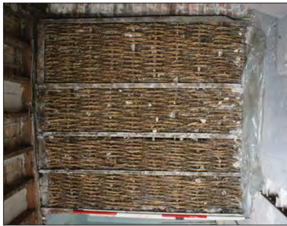
Plate 46. Room 5 First Floor. Rope and Plaster Partition Detailed Shot of Four Panels
