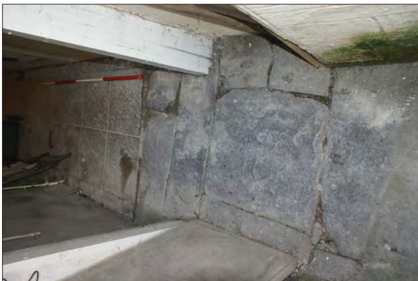
Plate 67. Slate Floor Slabs in Passageway Between 21 & 23 High Street
