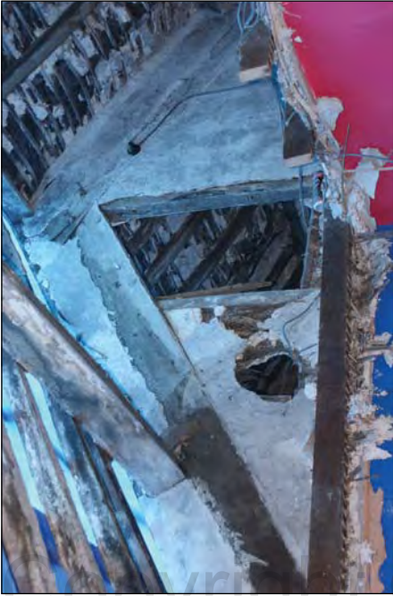
Plate 13. Roof Space Above Room 1. Divides Level in Half. Constructed of Twisted Rope and Plaster. Shows Attic Space
