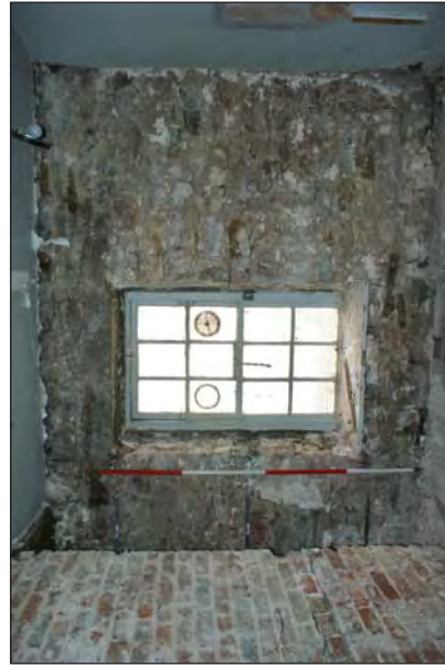
Plate 51. Room 6 First Floor. Gable Wall Showing Partition With Room 5 and Edge Of Fireplace
