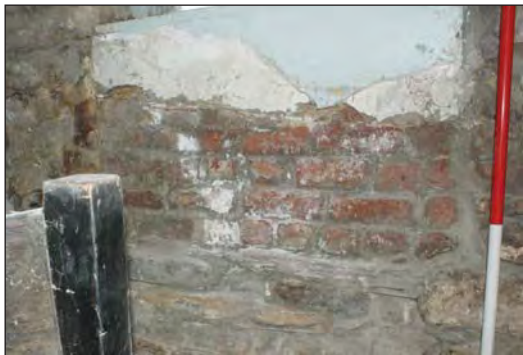
Plate 64. Blocking Below Window on First Floor Landing
