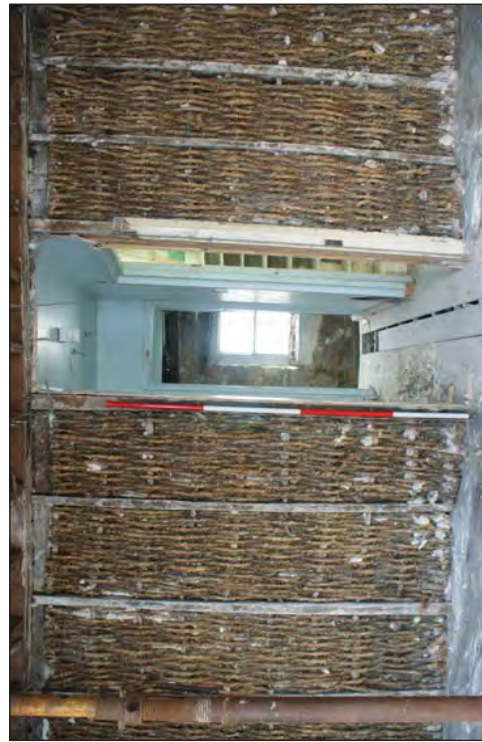
Plate 45. Room 5 First Floor. Rope and Plaster Partition to the Right Hand Side of Door
