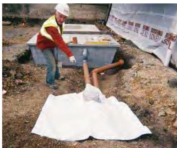
With rainwater – use separate pipe
