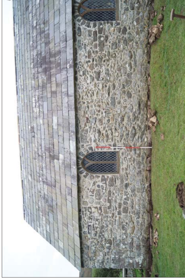
Plate 12. Northern Elevation Showing Patching with Smaller Stone Between Chancel and Nave and Remains of Lancet Window
