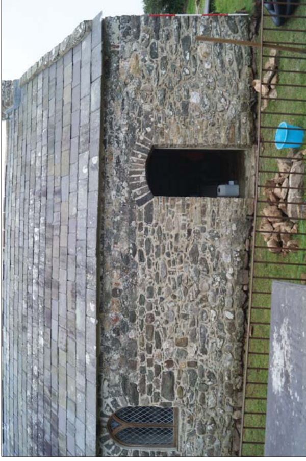
Plate 11. St. Mary's Church, Penllech. Northern Elevation Note Medieval Stonework at Base of Wall
