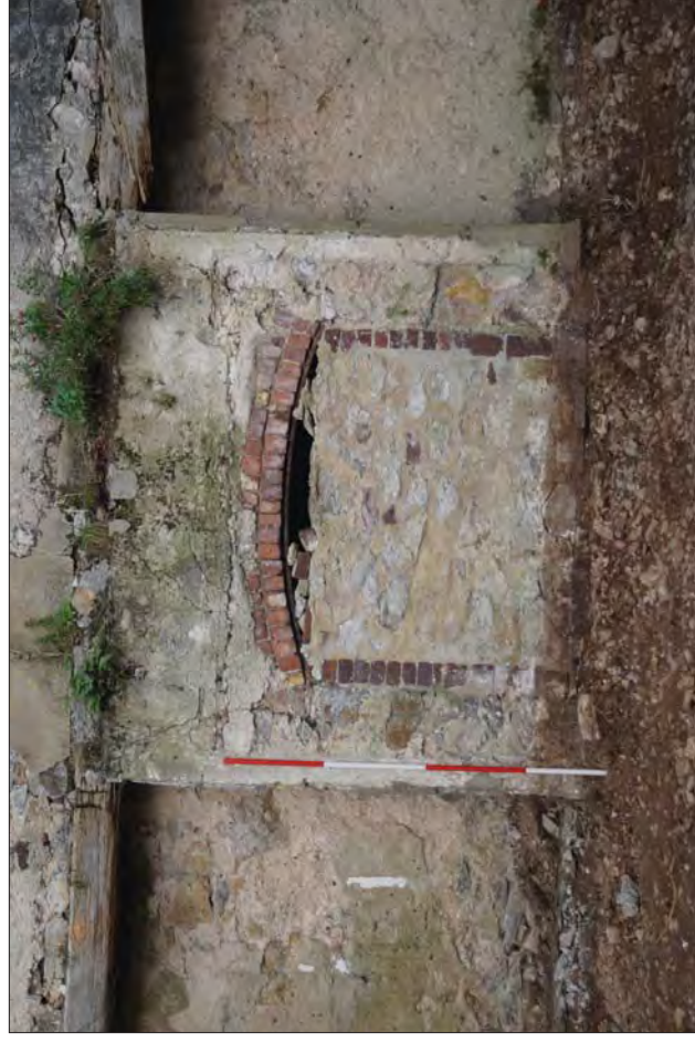
Plate 18. Detail of Blocked Fireplace at Ground Floor Level
