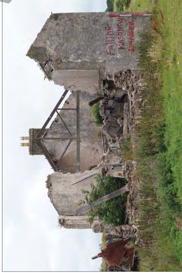
Plate 3. South-West Facing Gable Elevation Showing Collapsed Bell Tower
