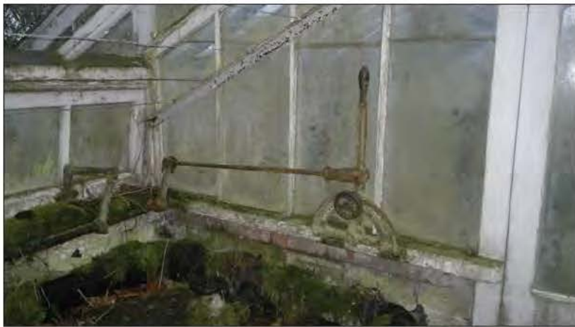
Plate 81. Central Greenhouse Interior Detailing Mechanism for Opening Ventilation Flaps. Photograph Source Mr. M Herman
