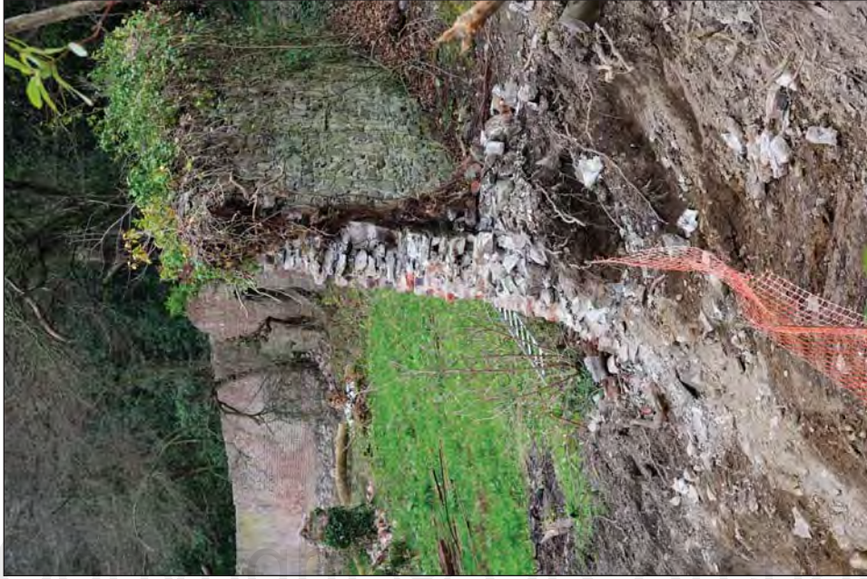
Plate 19. North-Western Garden Wall. Note The Differences Between This Wall and the Wall to the East of the Outbuilding. This Wall Has No Heating Ducts
