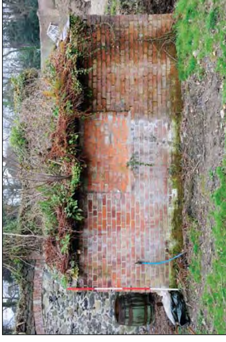
Plate 116. Bothy Side Elevation. Note Bricked-up Window
