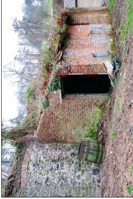
Plate 115. Bothy Front & Side Elevations. Note Blocked Walled Garden Entrance
