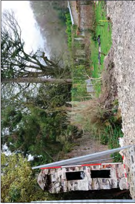
Plate 7. Garden Walls North-Eastern Section. Shows Cross-Section of Wall Interior With Heating Ducts
