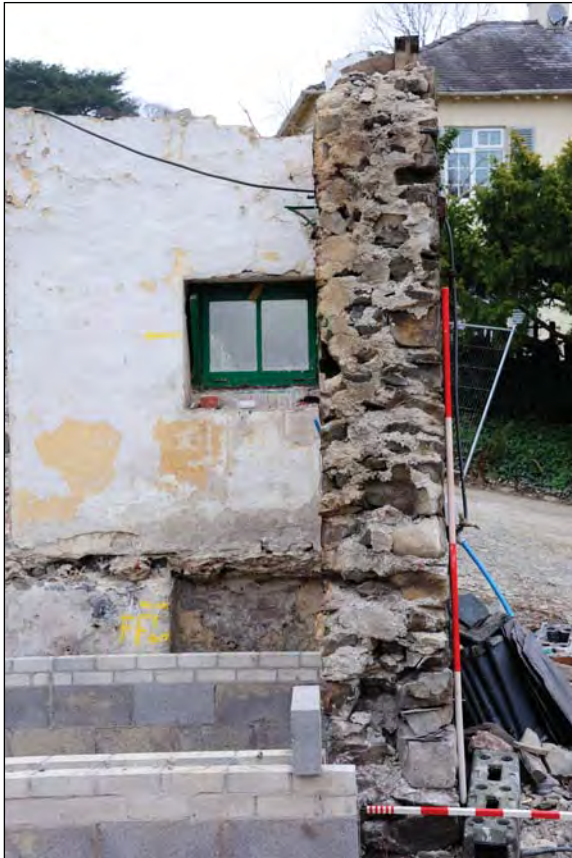
Plate 56. Outbuilding Rear Elevation Showing Stone Wall Construction
