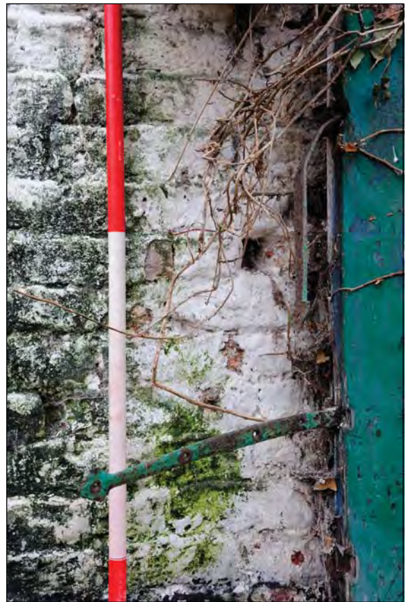
Plate 105. Iron Work on Stable Door-frame
