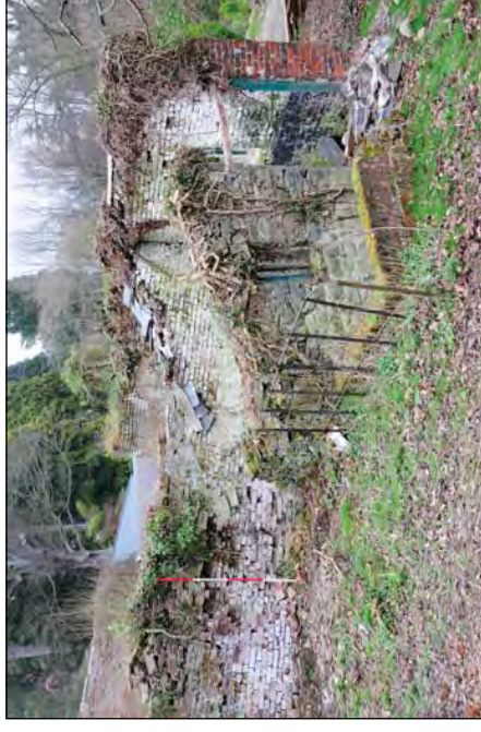
Plate 103. Stable Building Front Elevation and Roof Line. Note that in this Instance as it is the Outer Face of the Walled Garden Which Would be Visible and is made of Brick
