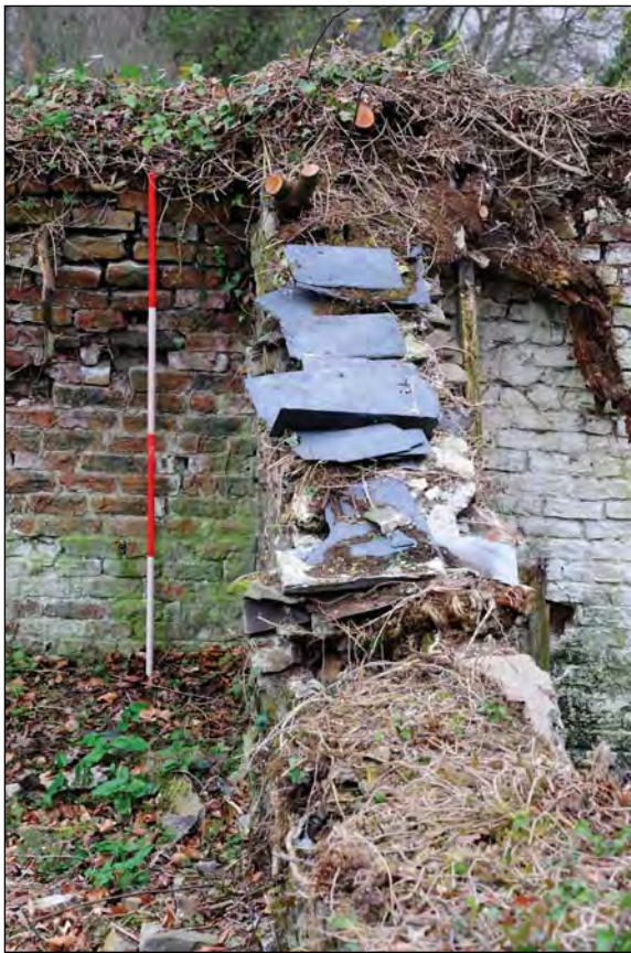
Plate 104. Stable Building Rear Wall and Roof Line with Surviving Slates.
