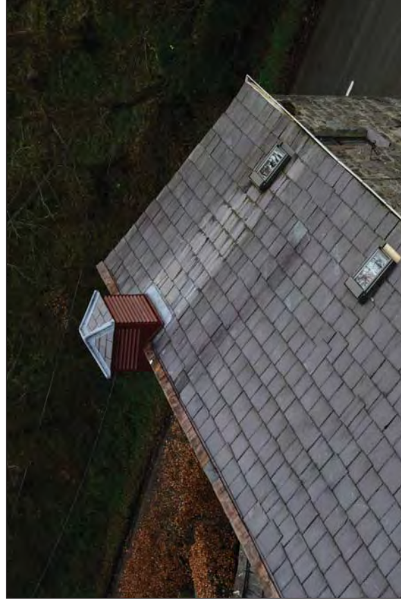
Figure 46. Slate Roof With Slatted Wooden Cupola Roof Vent (Largely Reconstructed) Serving as Evidence of Use as Corn Drying Kiln
