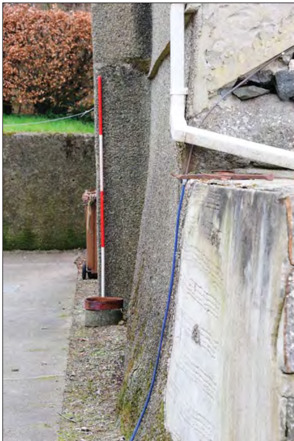
Figure 47. Rear of Mill/Kiln Structure. Note Splaying of Rear Elevation at Base of Wall
