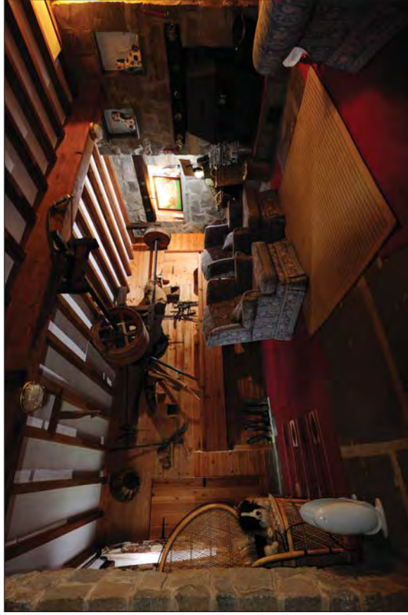
Figure 57. Ground Floor of Mill Showing Hurst Frame Boarding and the Iron Shaft/ Wooden Pulley System Belonging to the Sack Hoist
