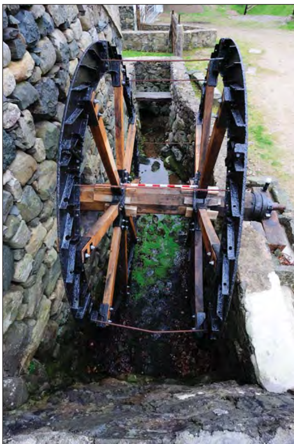
Figure 49. Waterwheel and Wheelpit. Possibly Pre-dating the Mill Structure
