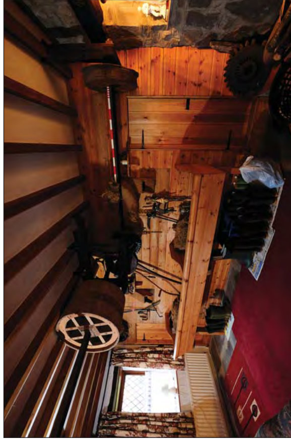
Figure 57. Ground Floor of Mill Showing Hurst Frame Boarding and the Iron Shaft/ Wooden Pulley System Belonging to the Sack Hoist
