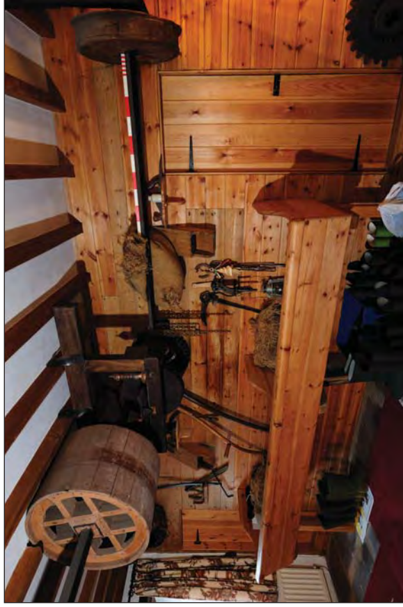
Figure 58. Ground Floor of Mill Showing Hurst Frame Boarding With Associated Trough and Flour Chutes
