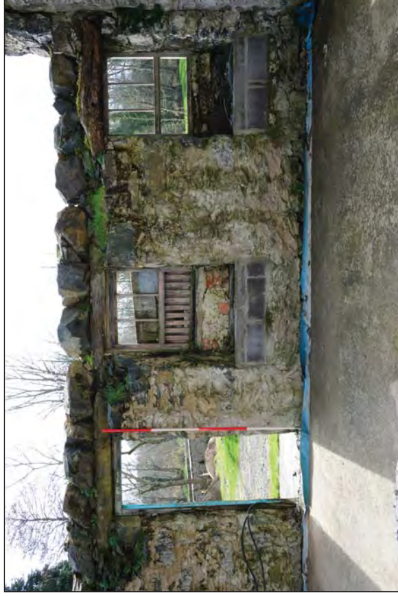
Figure 92. Interior View of Front Elevation of Miller's House Detailing Change in Window Heights
