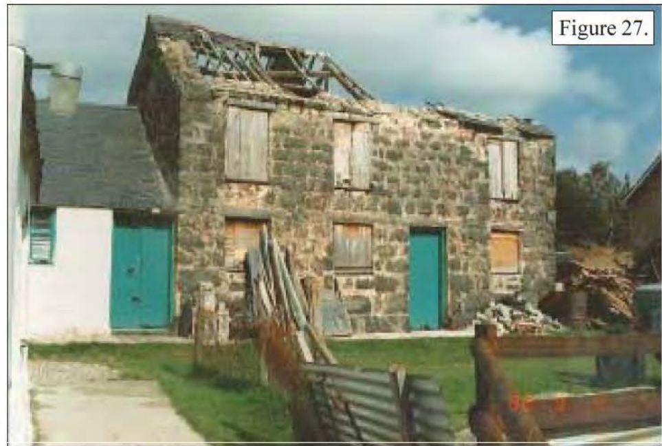
Figures 26 & 27. Photographs Taken of the Miller's House & Mill in the Late 1980's Following the 1984 Earthquake. Note The Large Crack in the Masonary
