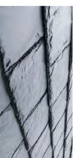
Natural Slate Roof
