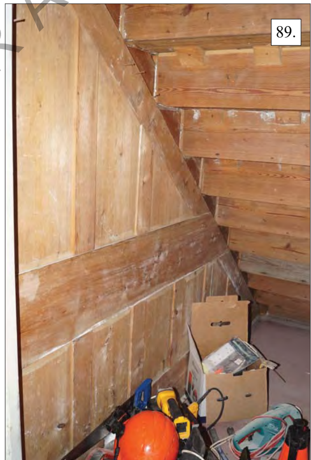
Plates 86 - 89. Wern Wen Farmhouse - Ground Floor - Hallway (Rm 3) Victorian Staircase and Brick Remodelling to Create Hallway, Storage Below Stairs
