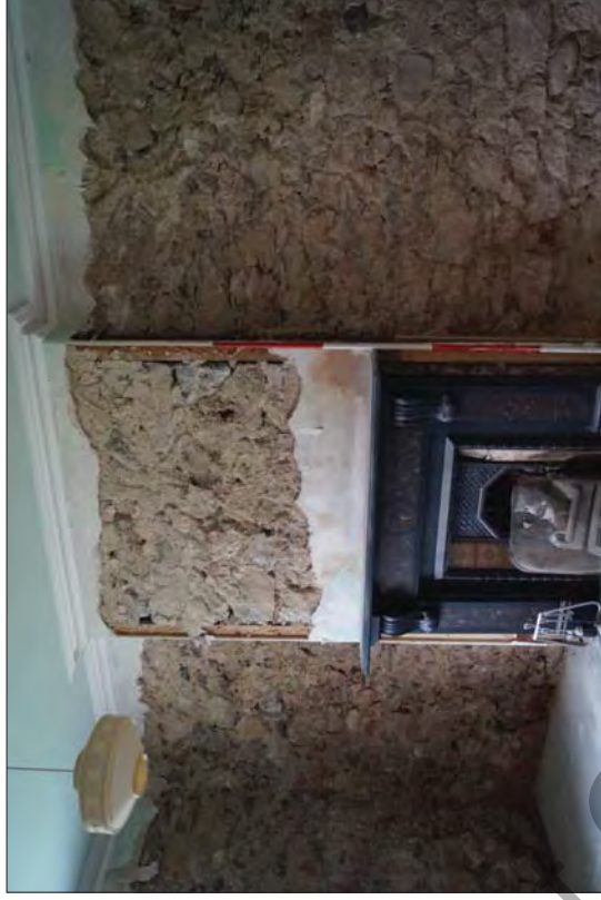
Plate 91. Farmhouse - Ground floor - Room 4 - Surviving Victorian Fireplace (Note Widening to Fit Fireplace)
