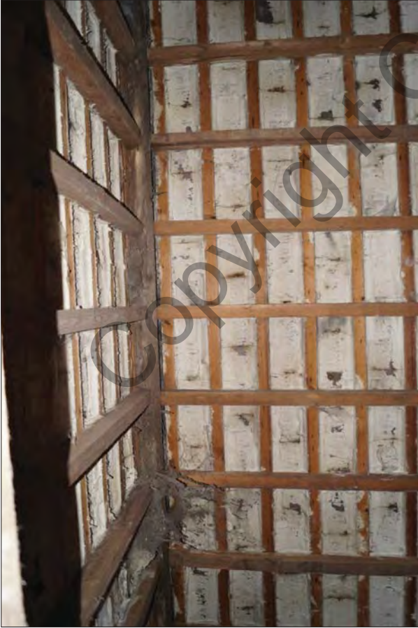
Plate 115. Farmhouse - First Floor - Room 6 - Lathe & Plaster Roof
