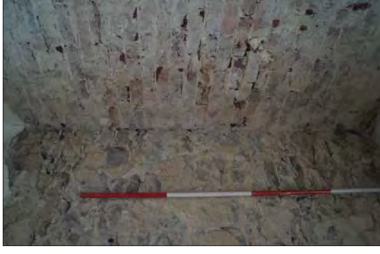
Plate 98. Details of Join Between Brick & Stone
