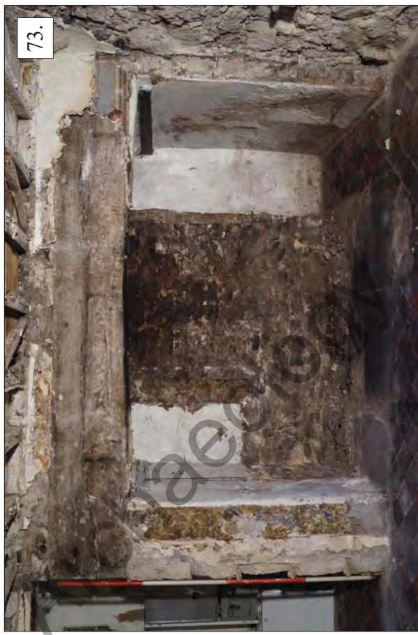
Plates 72 - 73. Wern Wen Farmhouse - Ground Floor - Living Room (Rm 2) Showing Large Inglenook Fireplace
