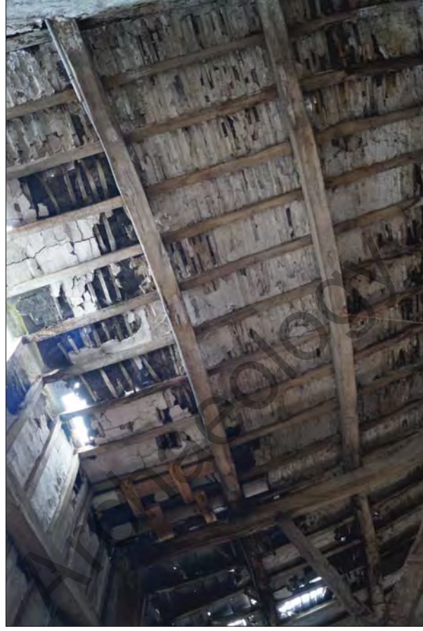
Plate 48. Wern Wen Barn Roof Structure Showing Pegged Joint
