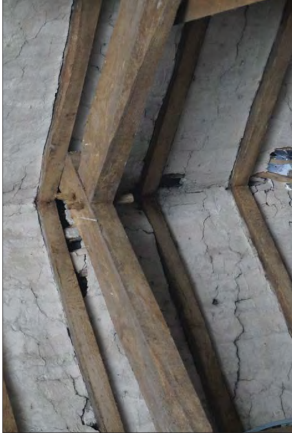
Plate 48. Wern Wen Barn Roof Structure Showing Pegged Joint
