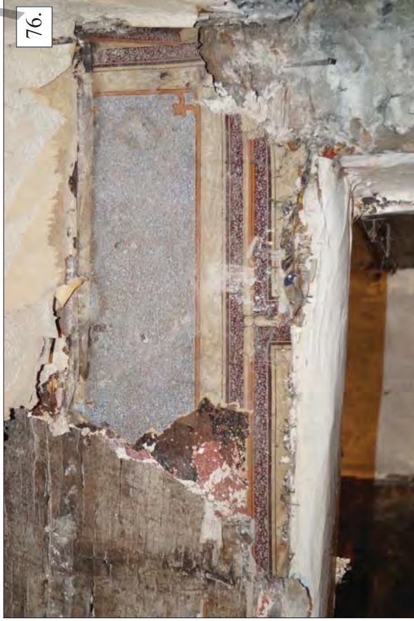
Plates 76 - 77. Wern Wen Farmhouse - Ground Floor - Living Room (Rm 2) Showing Early Handpainted Wallpaper and Axial Beam
