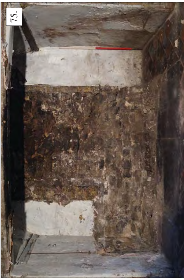
Plates 74 - 75. Wern Wen Farmhouse - Ground Floor - Living Room (Rm 2) Large Inglenook Fireplace Showing Flooring & Hook Rows
