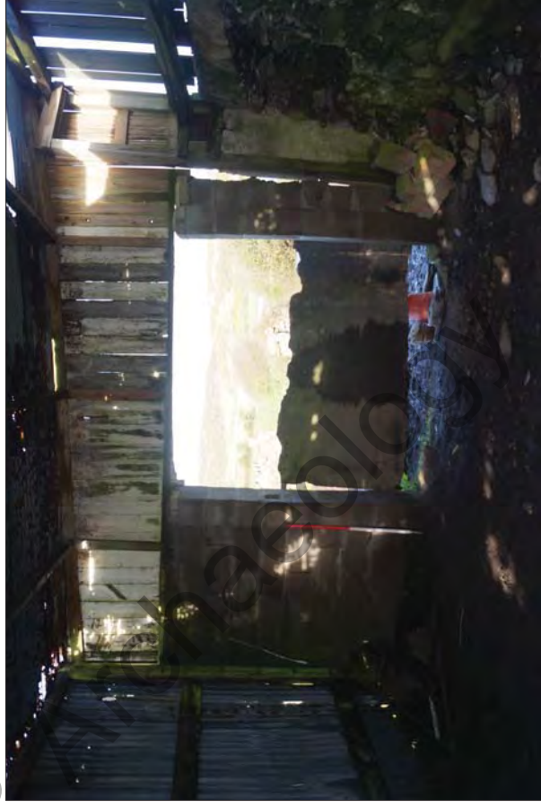
Figure 37. Interior of Building 5 - Barn. Showing Earlier Boundary Wall Incorporated into Structure
