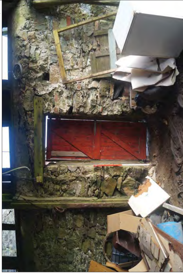
Figure 38. Interior of Building 5 - Barn. Showing Earlier Boundary Wall Incorporated into Structure
