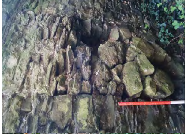
Plate 28a & b. Rear Elevation of Building 7 Showing Blocked Opening
