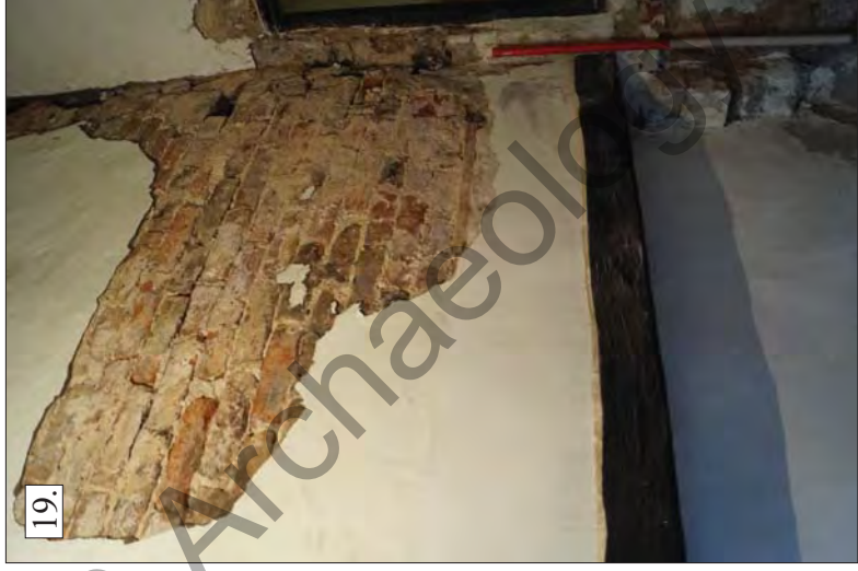
Plate 18. Front (North-Eastern) And Gable (South-Eastern) Elevations Following Removal Of Plaster. Demonstrates That House has not Been Constructed By Simply Adding the Front Wall And a Roof
