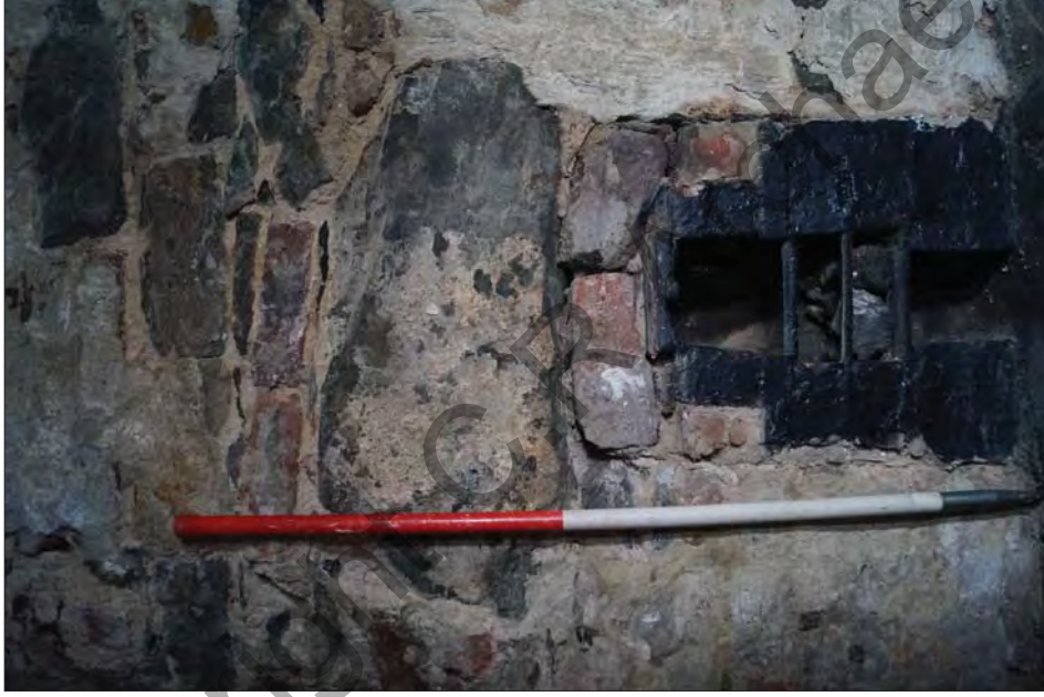
Plate 21. Fireplace and Chimney Breast Following Removal of Plaster
