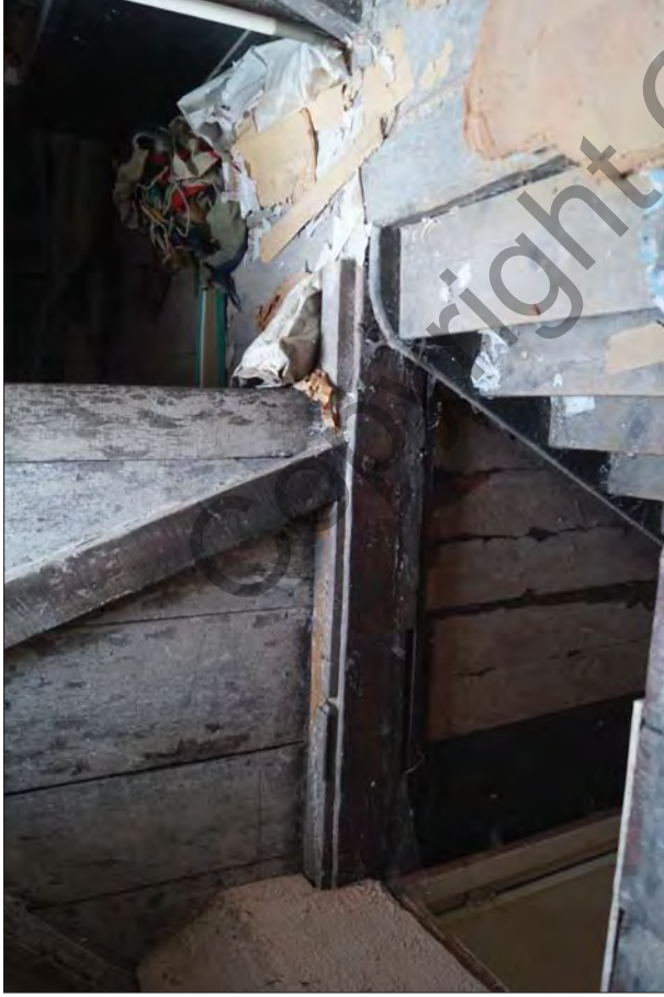
Plate 23. 11 Lower Gate Street, Attic Level Facing Towards North-Western Gable Showing Wooden Room Division
