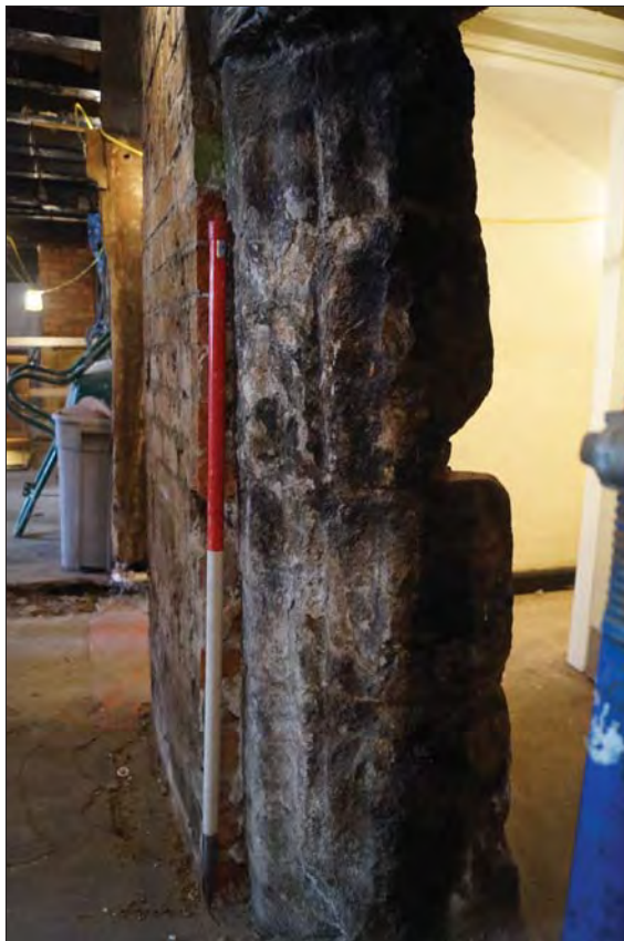
Plate 11. Fireplace Jamb Following Stripping Out Works
