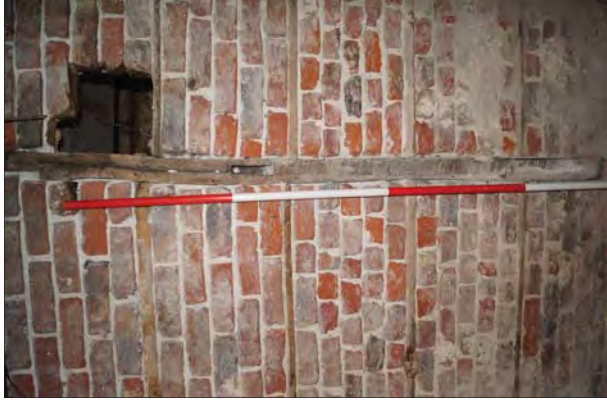
Plate 27. Mortice Joint in Timber Framing
