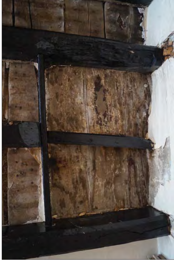
Plate 37. Ceiling Above Front Lounge Showing Position Of Earlier (Original?) Stairway to First Floor
