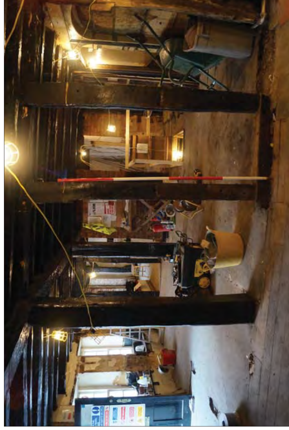
Plate 29. Timber Uprights of Internal Partition - Note Peg Holes in the Central and Right Hand Posts
