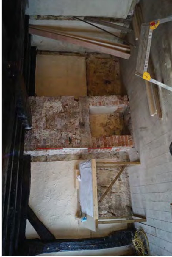
Plate 36. Late Georgian Brick Fireplace With Wooden Lintel Concealed Behind Later Render
