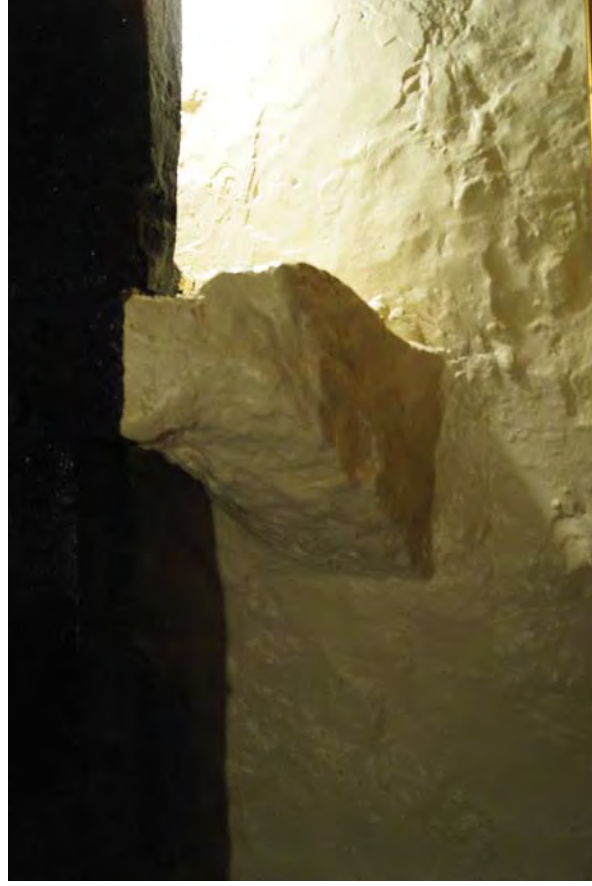
Plate 43. Corbel Supporting Head Beam
