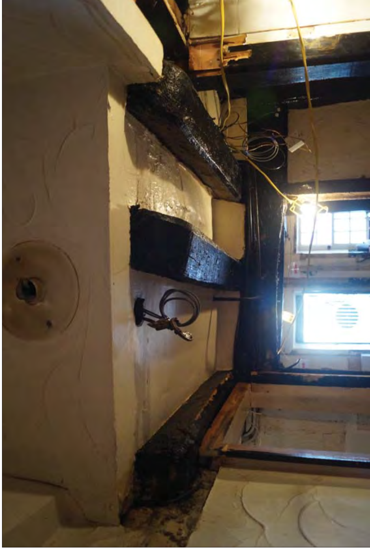
Plate 48. Three Projecting Jetty Joists in Area Behind Bar
