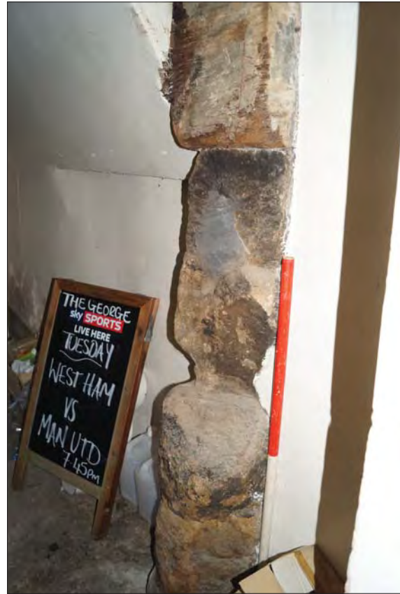
Plate 10. Fireplace Jamb Visible Prior to Stripping Out Works
