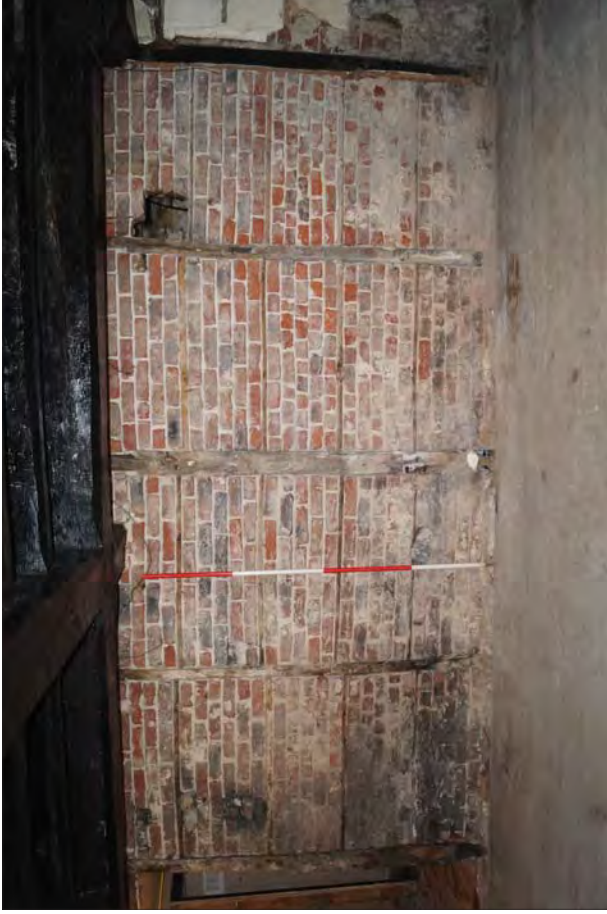
Plate 25. Timber Framed Partition Wall with Later Brick Nogging
