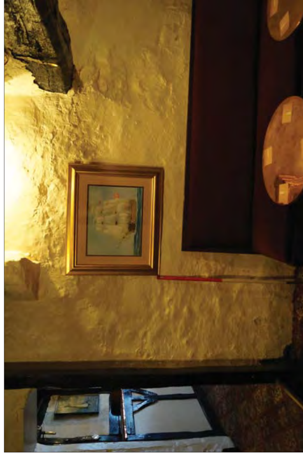
Plate 42. Stone Partition Wall and Corbel Supporting Head Beam
