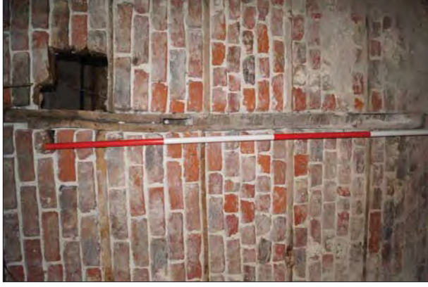
Plate 27. Mortice Joint in Timber Framing
