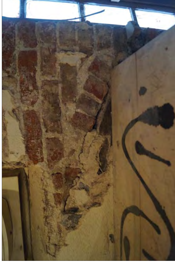
Plate 35. Brick Arch Detail Above Cellar Door
