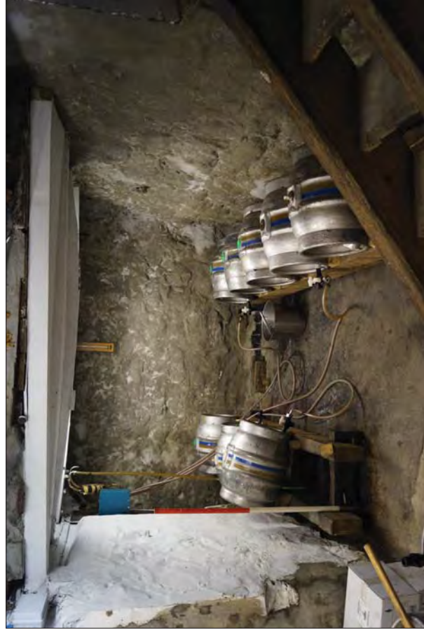
Plate 38. Cellar Drop from Bar Area Note Stepped Rough Stone Corbelling to Left Hand Side
