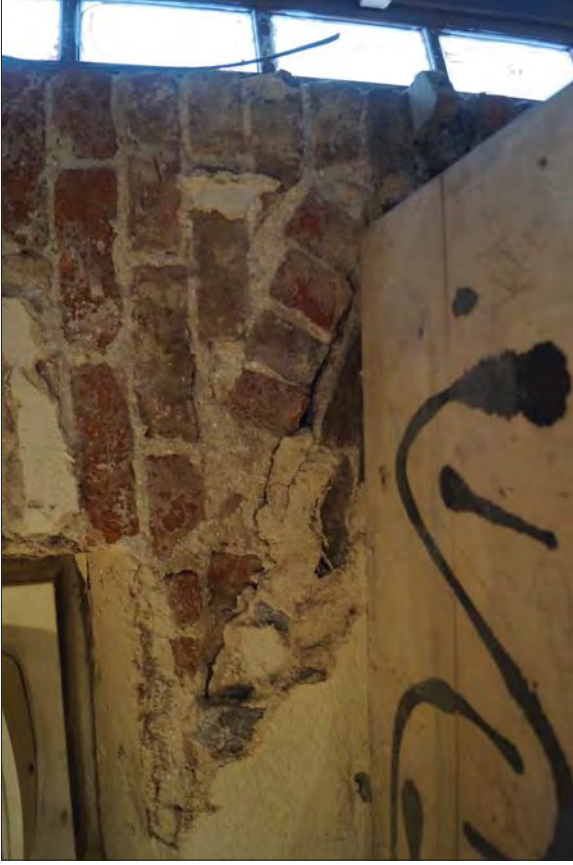
Plate 35. Brick Arch Detail Above Cellar Door
