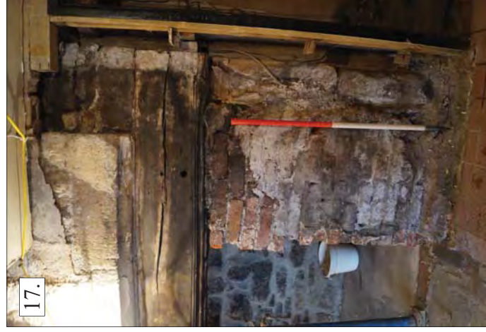
Plate 17. North-Western Jamb and Brick Infill. Note Peg Holes In Wooden Lintel
