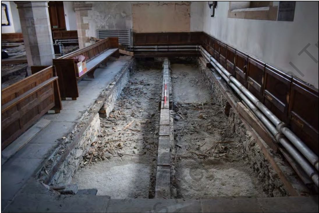
Fig. 2: The north aisle floor, showing the sleeper walls, from the east. CPAT 4679-0001
