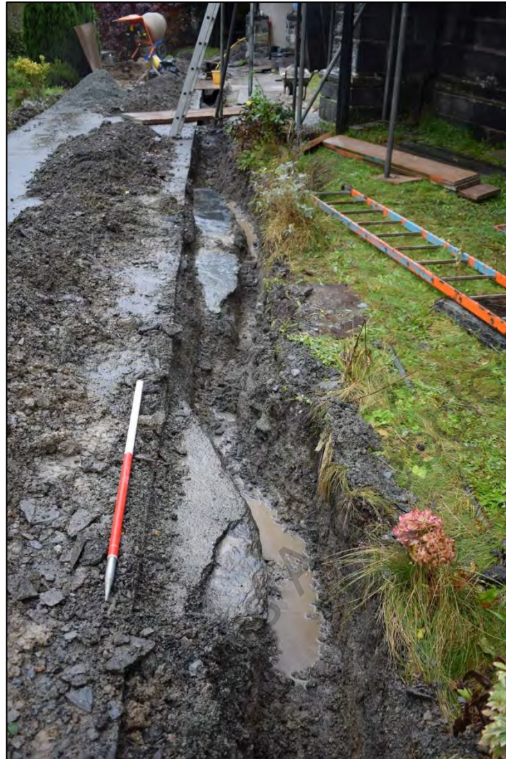
Fig. 25: Ledgers visible in the side of the trench for the waste pipe leading from the sewage treatment plant and following the line of the church path. CPAT 4679-0138
