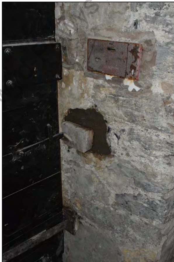
Fig. 23: The location of the (repointed) wooden drawbar slot on the external door of the chapel. CPAT 4679-0171
