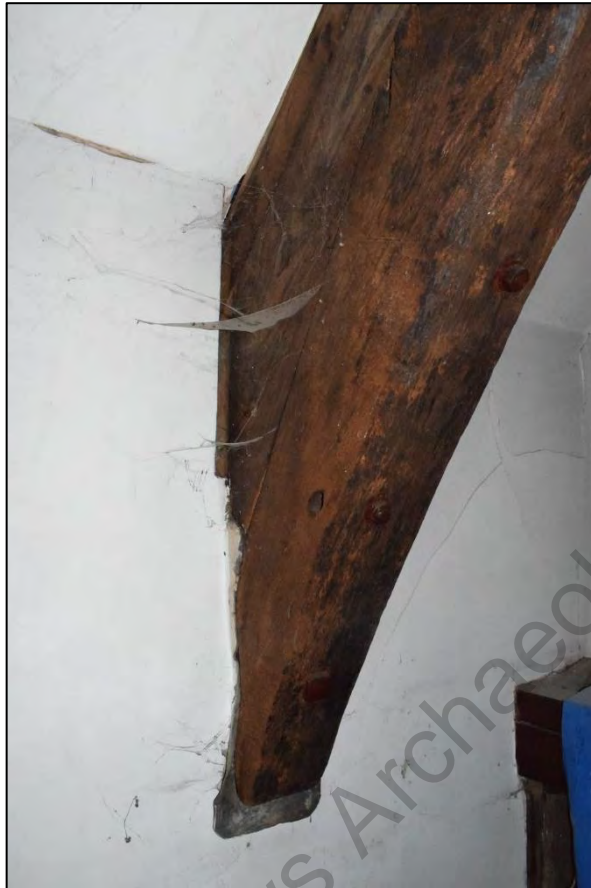
Fig. 17: The south side of the roof truss crossing the rood screen, showing bolted repair, from the north-east. CPAT 4679-0183
