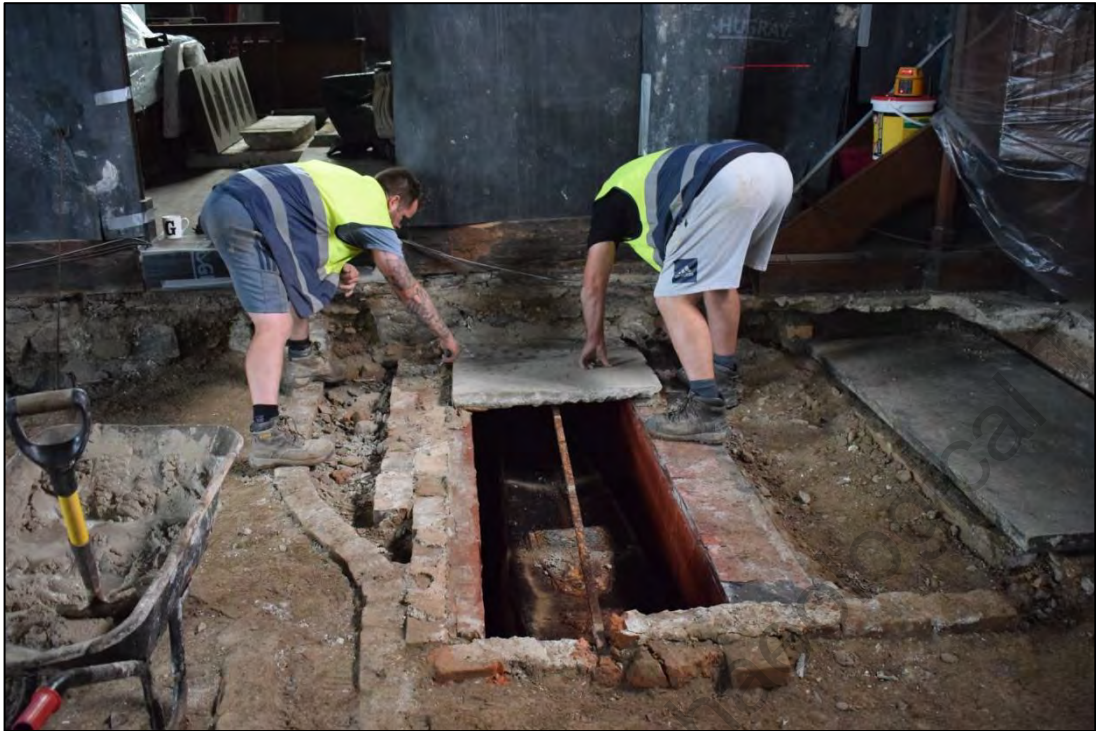
Fig. 12: The placement of the new capping stones over the north part of the vault. The ledger is in its lowered position. CPAT 4679-0105
