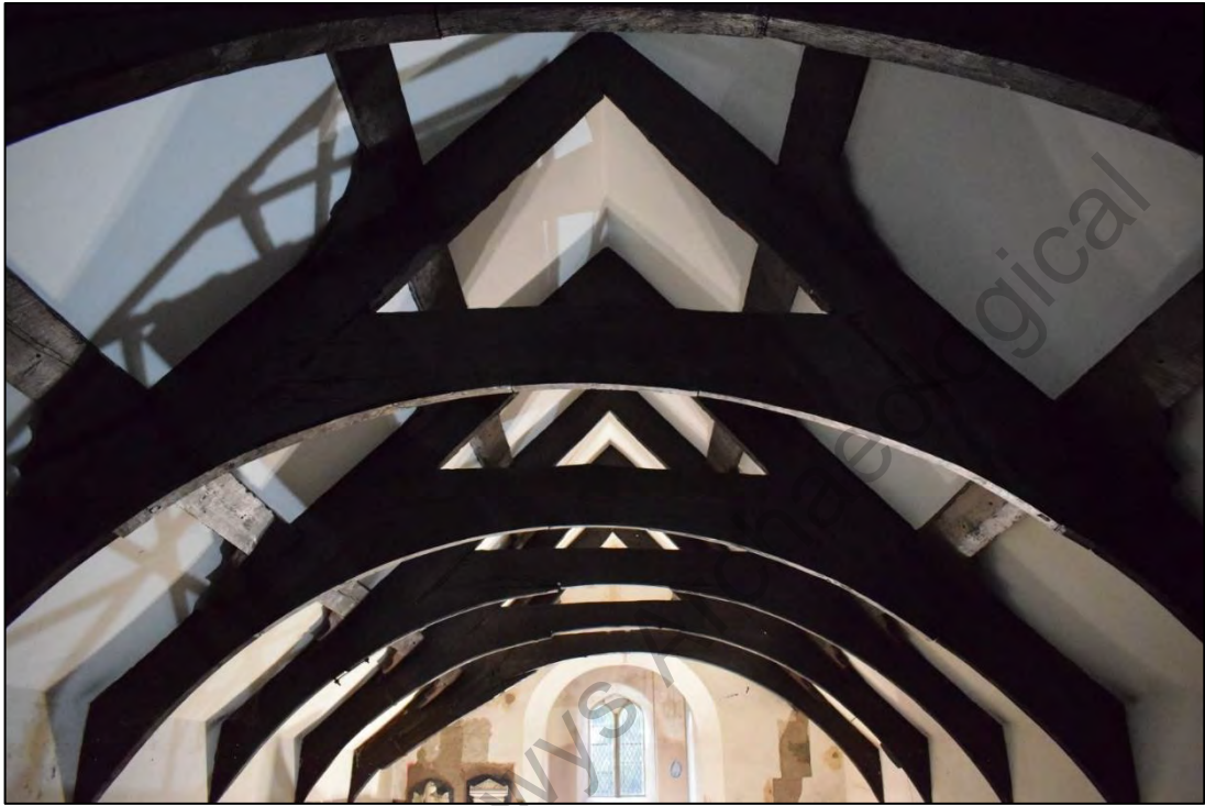
Fig. 16: The roof trusses in the nave taken from the top of the rood screen, from the east. CPAT 4679-0181
