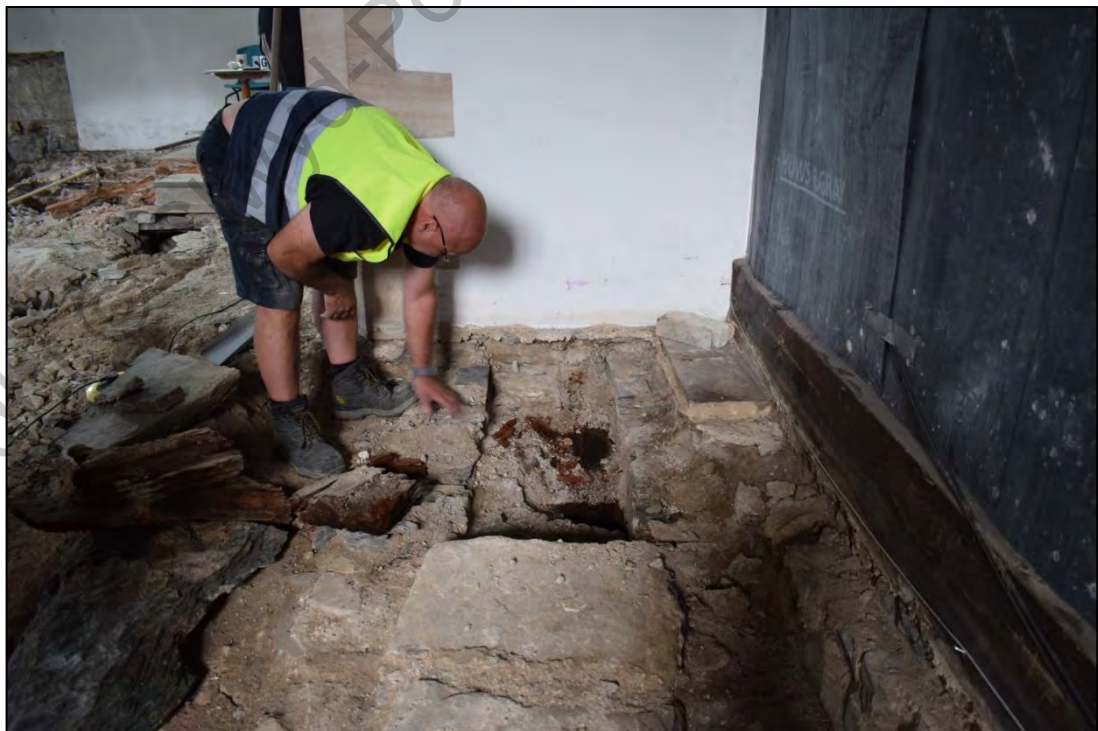
Fig. 9: The reduction in the height of the sleeper walls of Vault 2, prior to the setting in place of new covering slabs, from the south. CPAT 4679-0082
