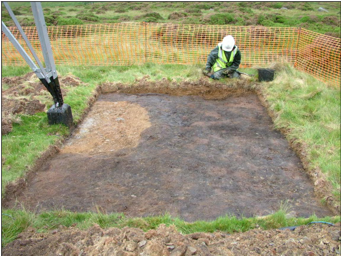
Fig. 3 View of the excavation with the west leg of tower AD26 visible; the backfill of the foundation excavation is readily apparent.
