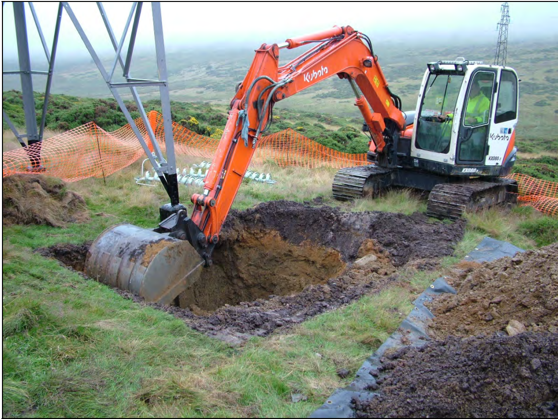
Fig. 6 Machining of the tower foundation investigations. Photo CPAT 3656-0021
