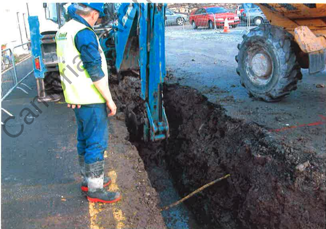
Plate 2: Conwy Quay works
