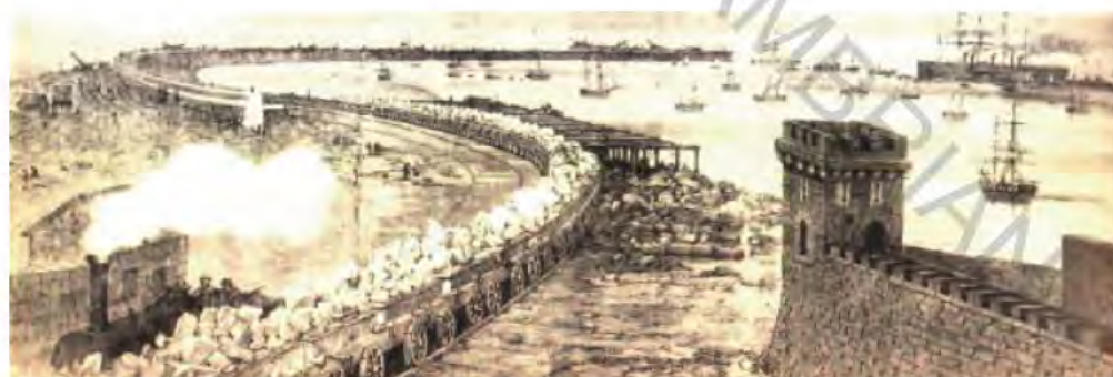
a) Breakwater under construction, c. 1858. Soldiers Point House screen wal in foreground.
