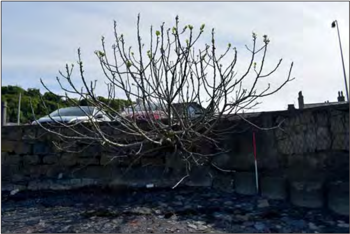
Plate 9: Fig tree growing from existing sea wall. View from north, scale:1m
