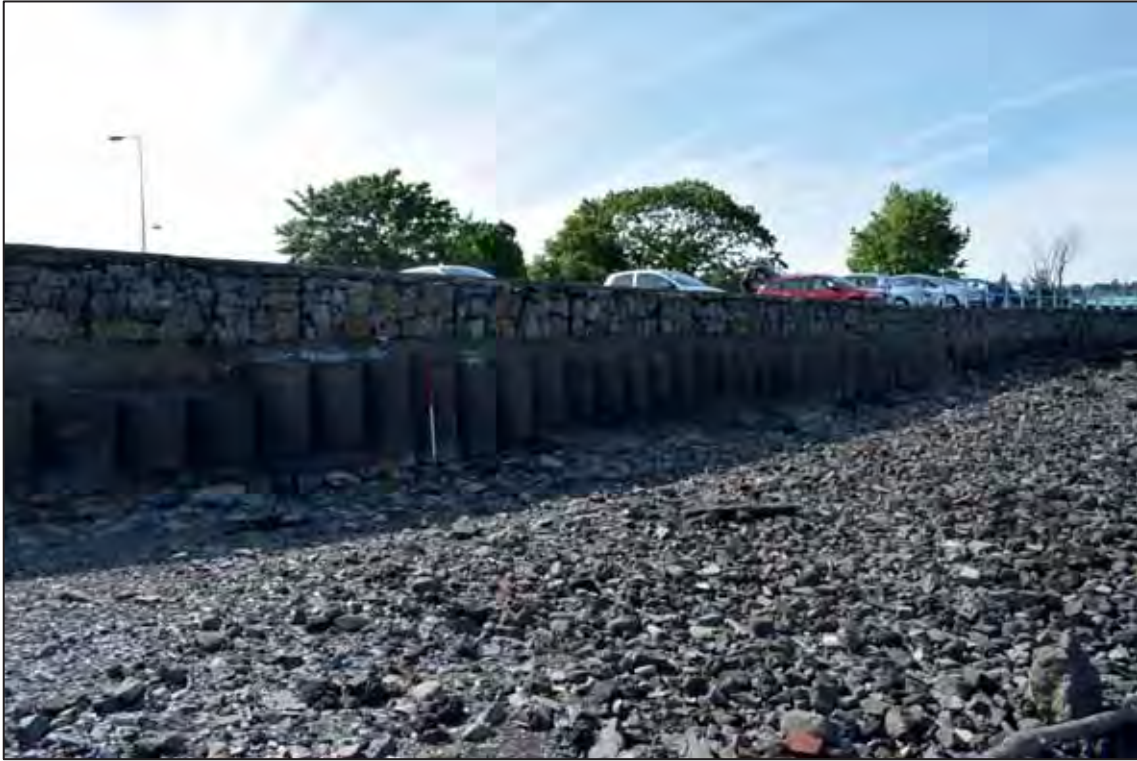
Plate 11: Anti-invasion devices re-used in existing sea wall. View from east, scale:1m
