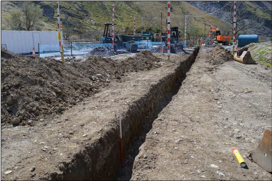
Plate 3: New sewer main trench from the east, scale: 1m
