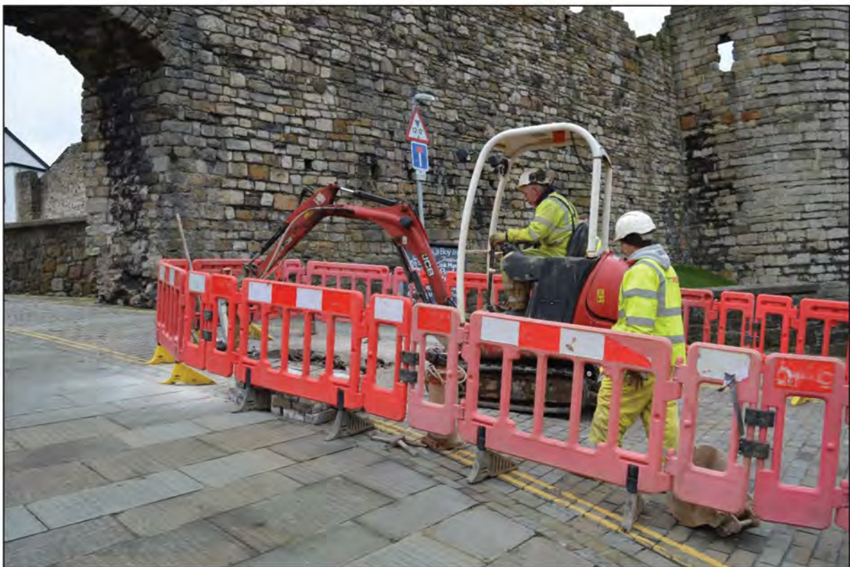
1. General view of works in progress, from the North-East
